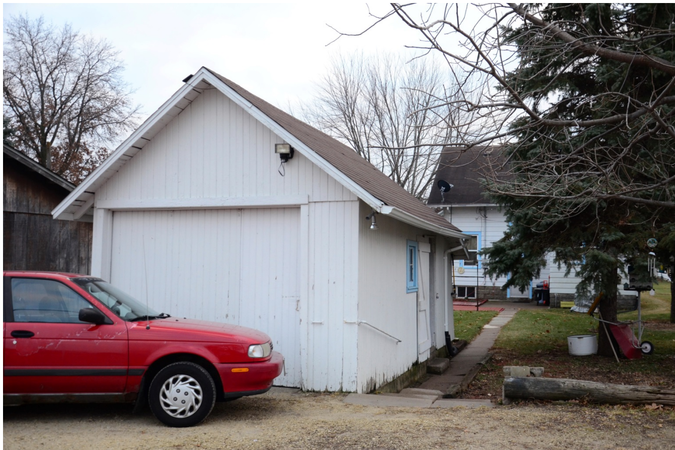
Photograph 92-00782-004 - Garage, looking southeast (December 2014)
