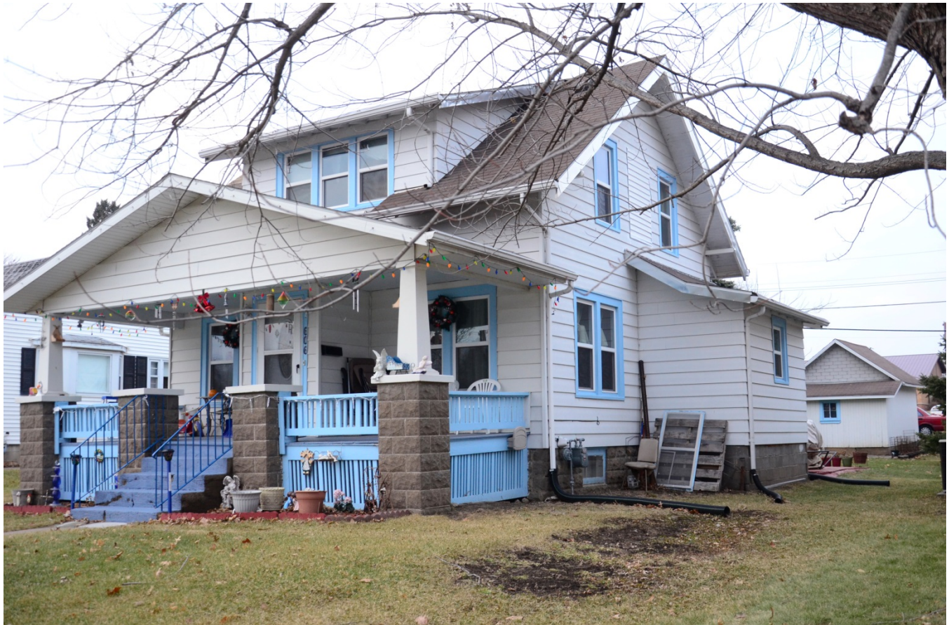
Photograph 92-00782-001 - House, looking northwest (December 2014)
