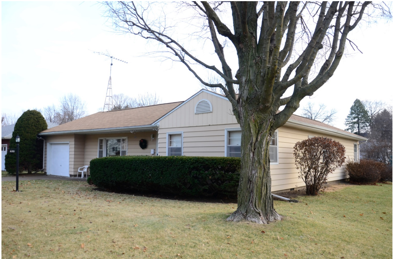
Photograph 92-00780-002 - House, looking southeast (December 2014)
