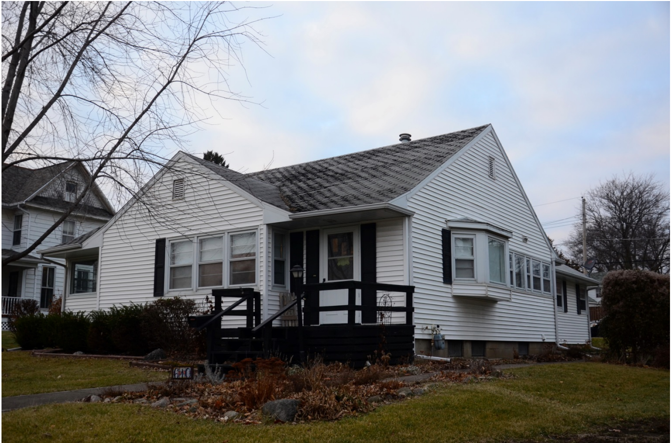
Photograph 92-00783-001 - House, looking northwest (December 2014)
