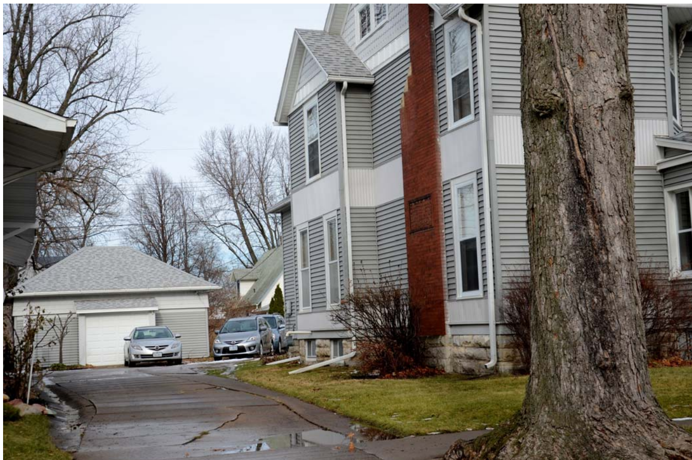
Photograph 92-00386-004 - Garage, looking north (December 2014)
