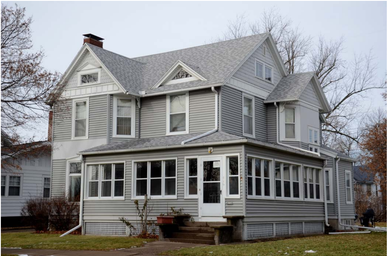
Photograph 92-00386-001 - House, looking northwest (December 2014)
