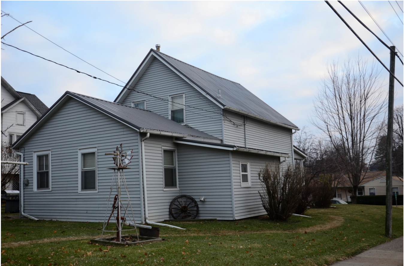
Photograph 92-00786-003 - House, looking southeast (December 2014)
