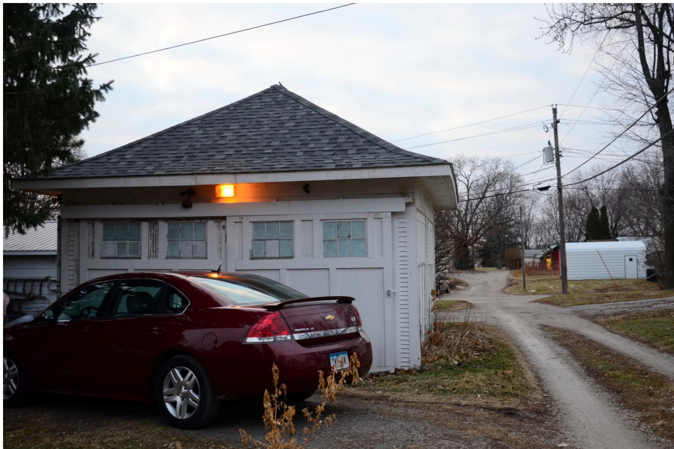
Photograph 92-00785-005 - Garage, looking west (December 2014)
