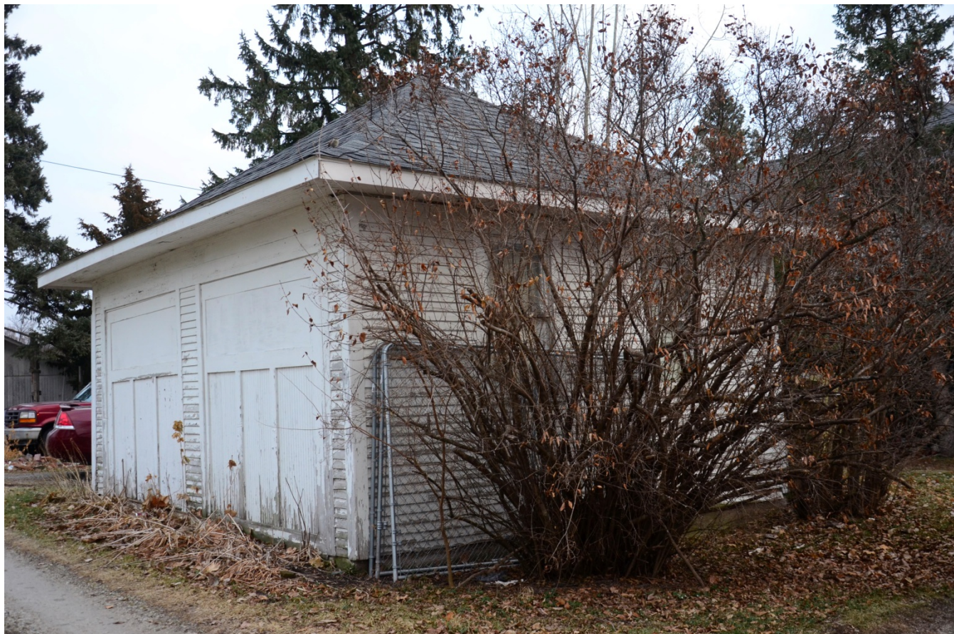
Photograph 92-00785-006 - Garage, looking west (December 2014)
