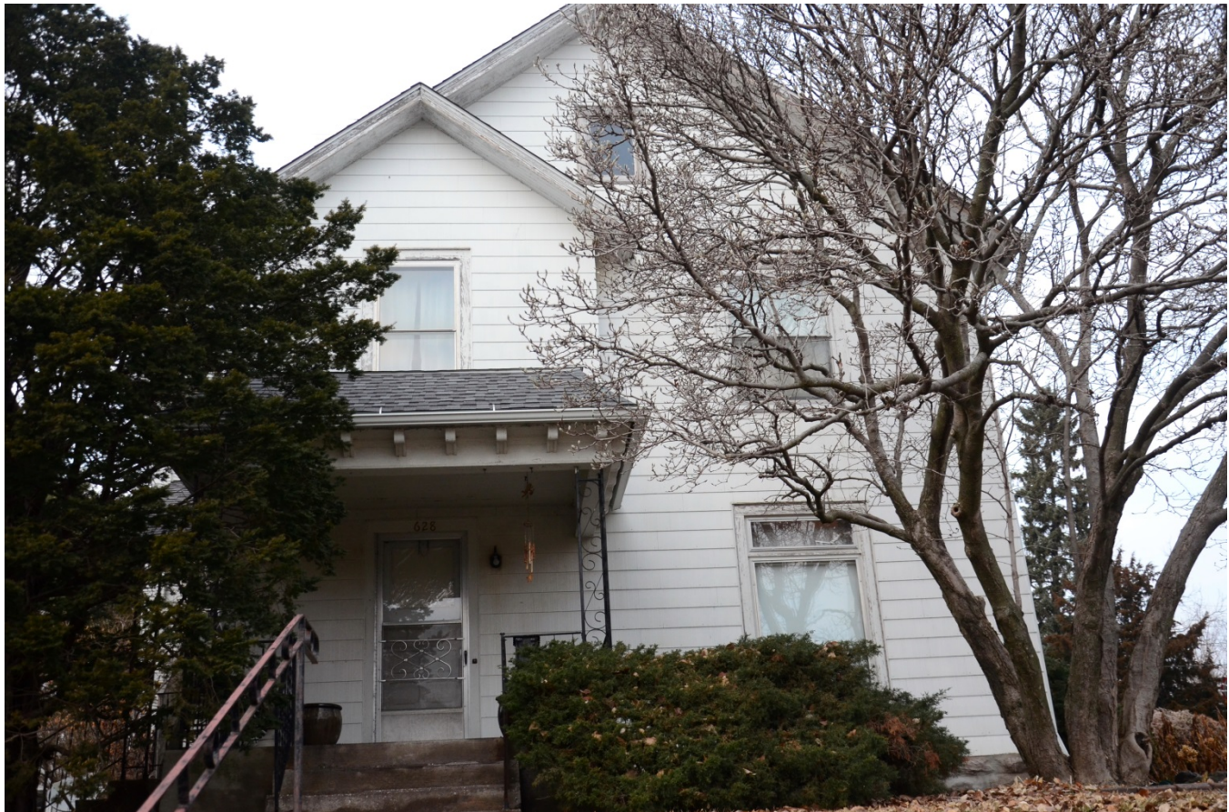
Photograph 92-00785-001 - House, looking north (December 2014)
