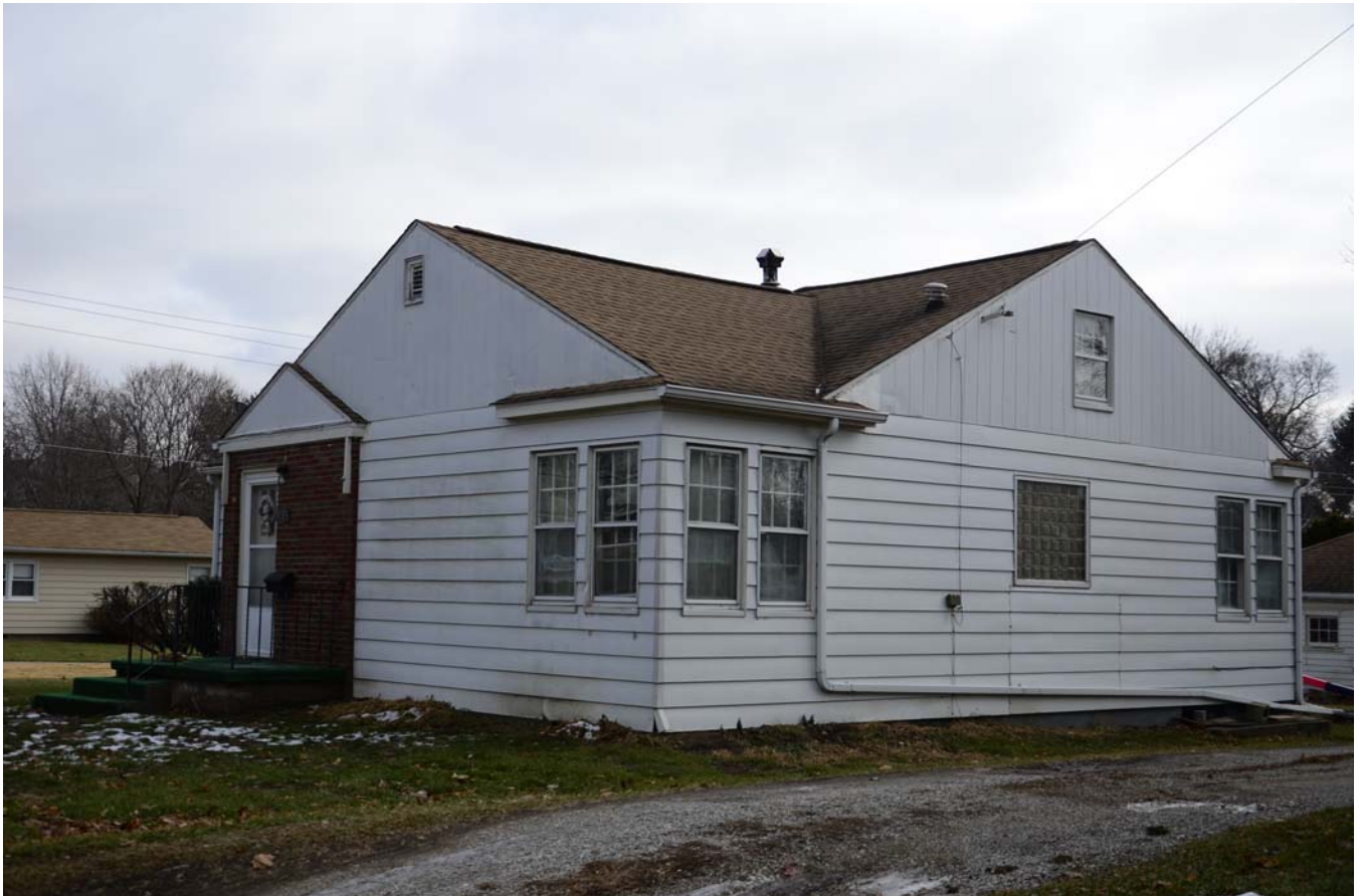
Photograph 92-00787-001 - House, looking southeast (December 2014)
