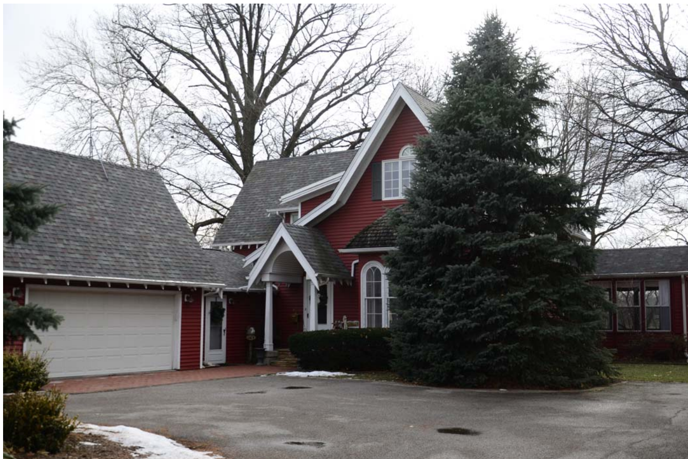
Photograph 92-00792-002 - House, looking southeast (December 2014)
