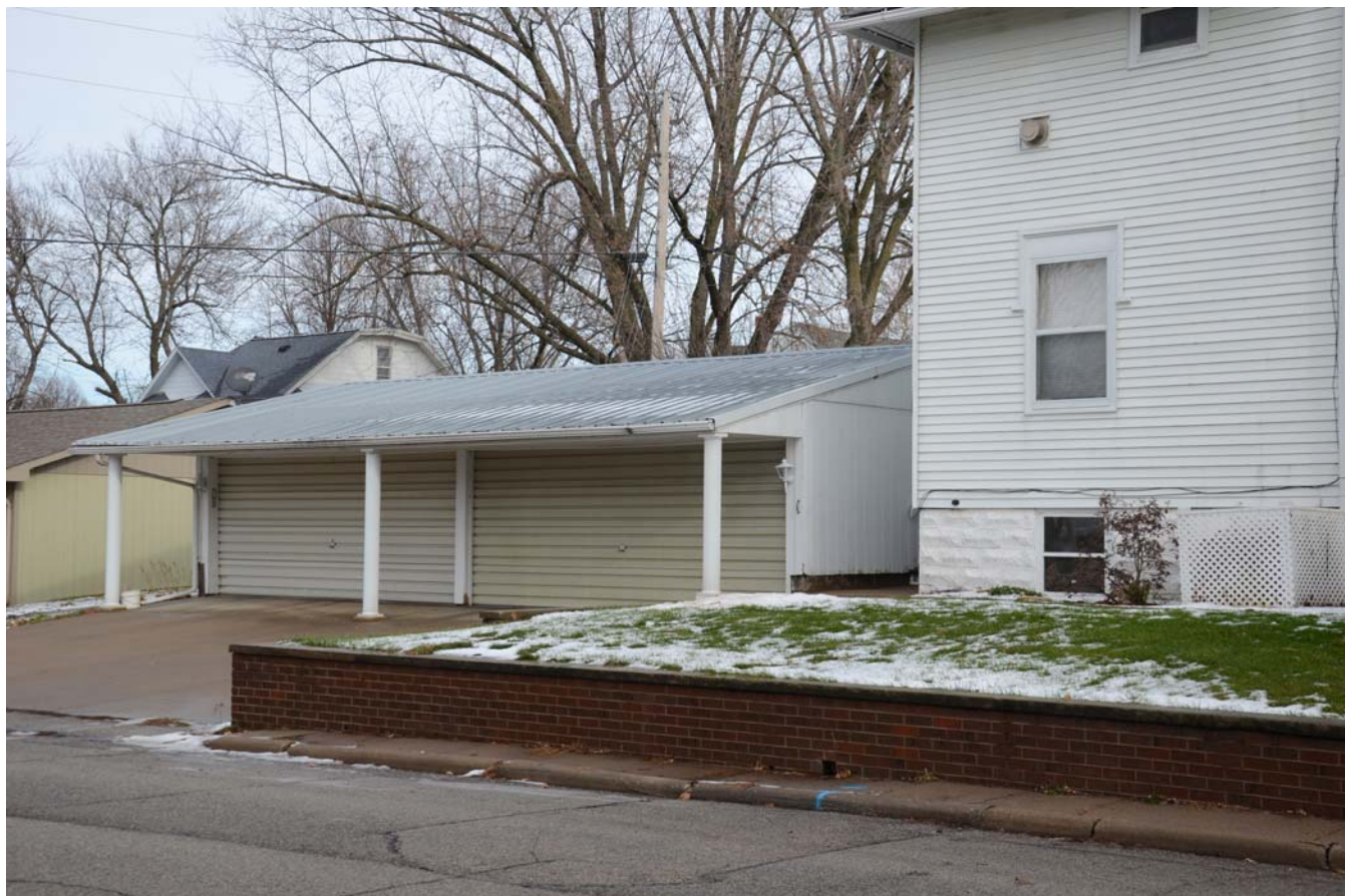
Photograph 92-00388-005 - Garage, looking northeast (December 2014)
