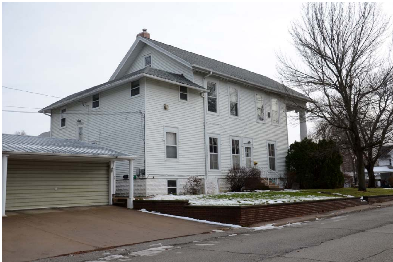
Photograph 92-00388-004 - House, looking southeast (December 2014)
