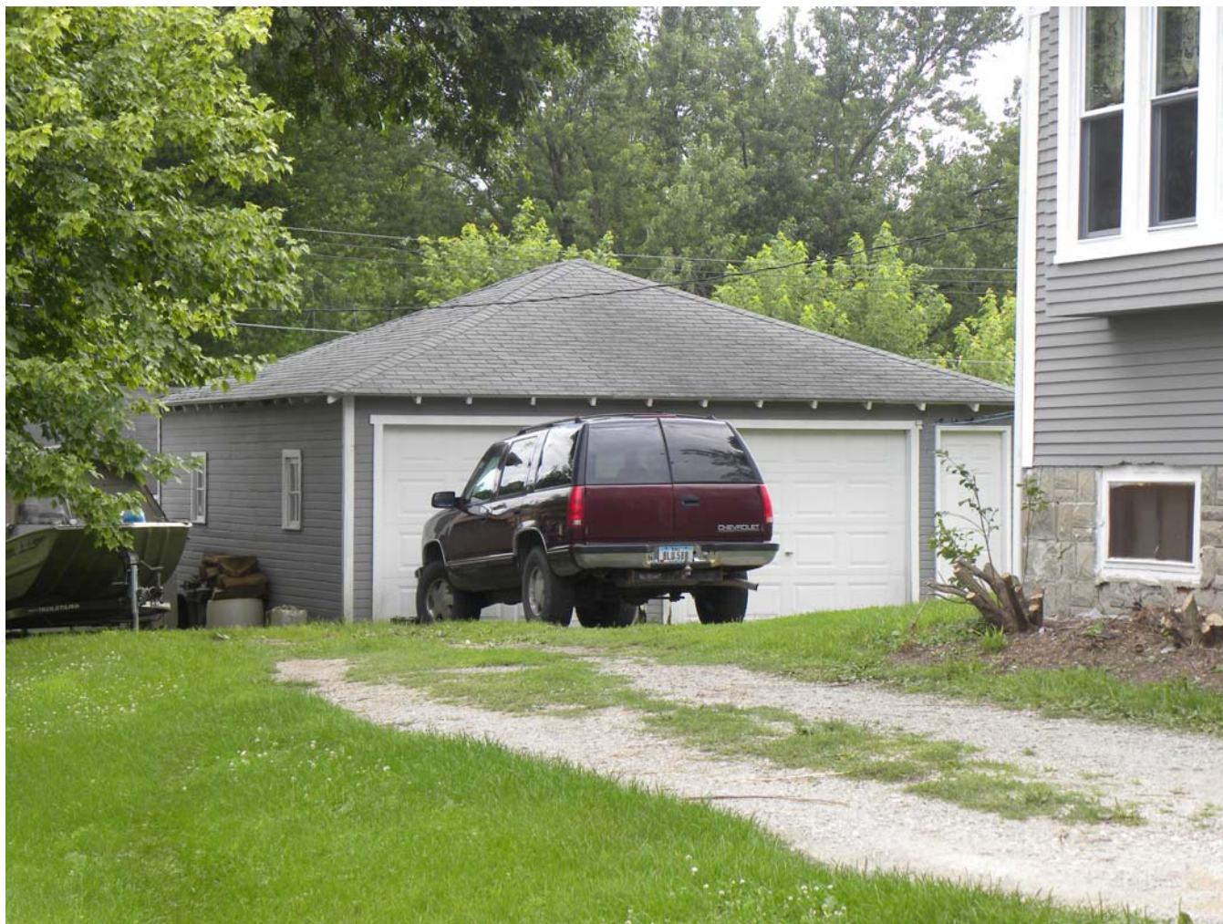
Photograph 92-00788-004 - Garage, looking southwest (July 2015)
