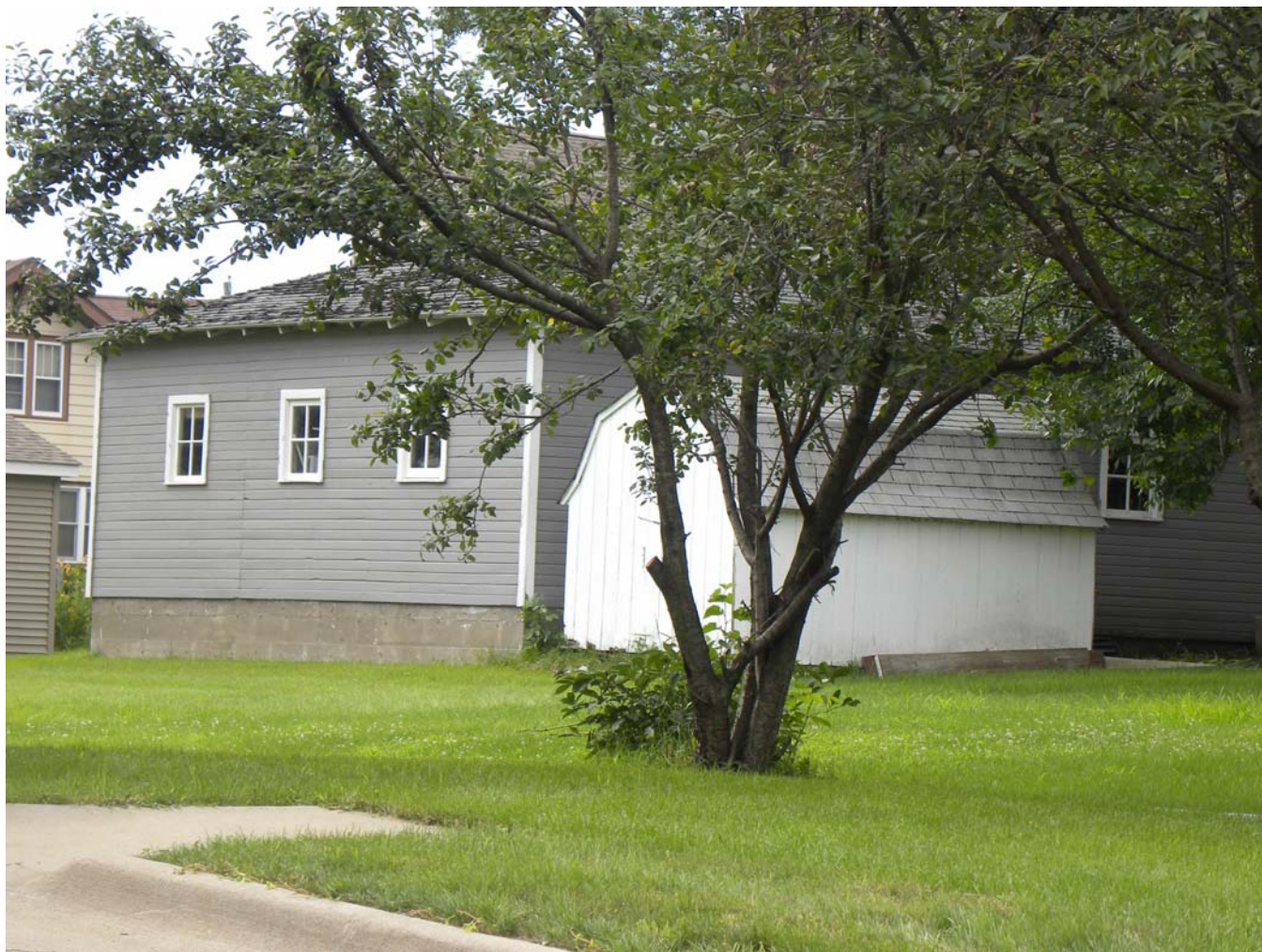
Photograph 92-00788-005 - Garage, looking northwest (July 2015)
