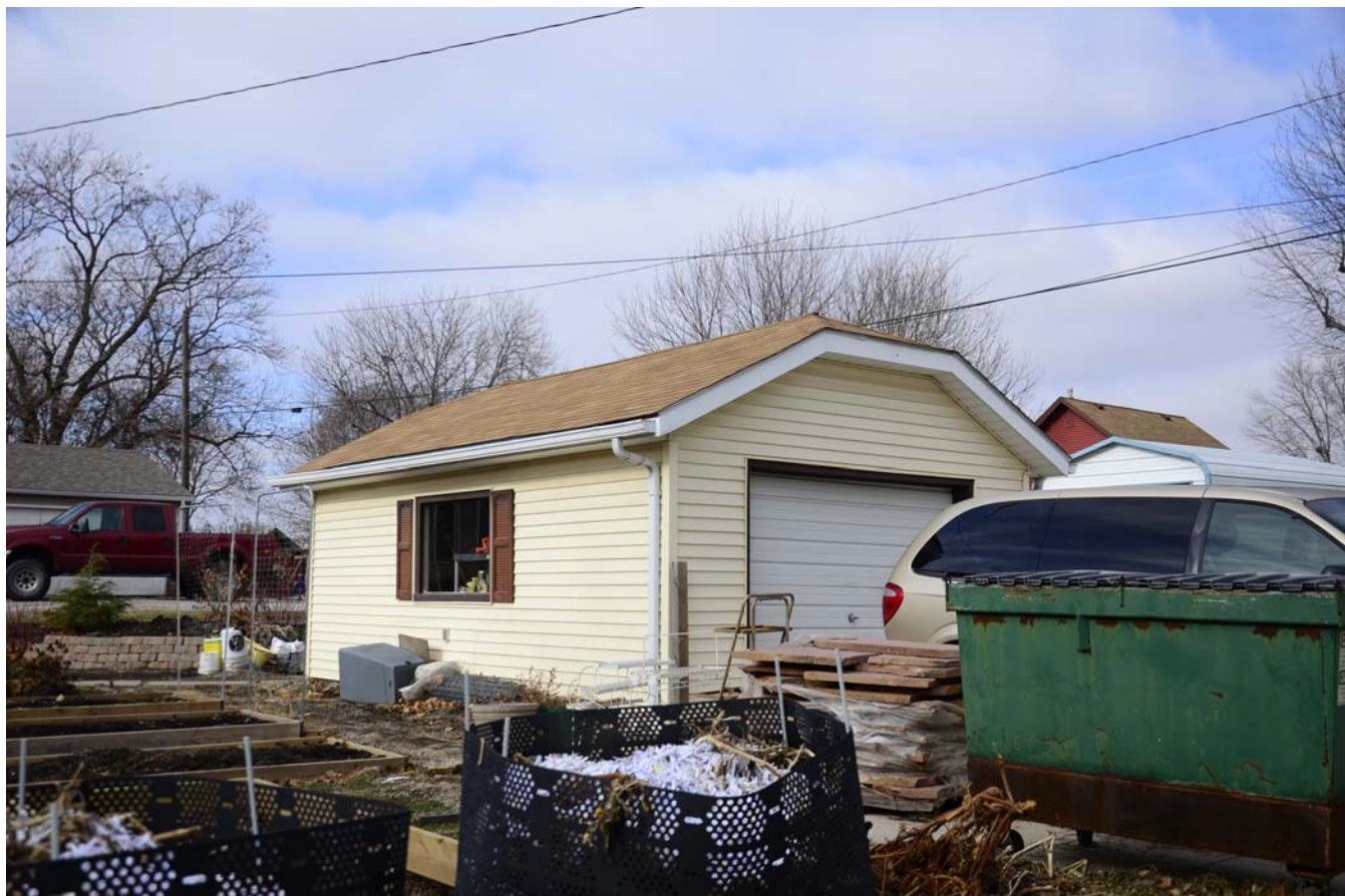
Photograph 92-00793-003 - Garage, looking northeast (December 2014)
