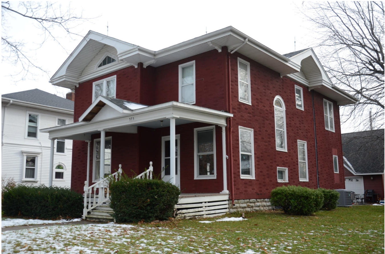
Photograph 92-00374-001 - House, looking southeast (December 2014)
