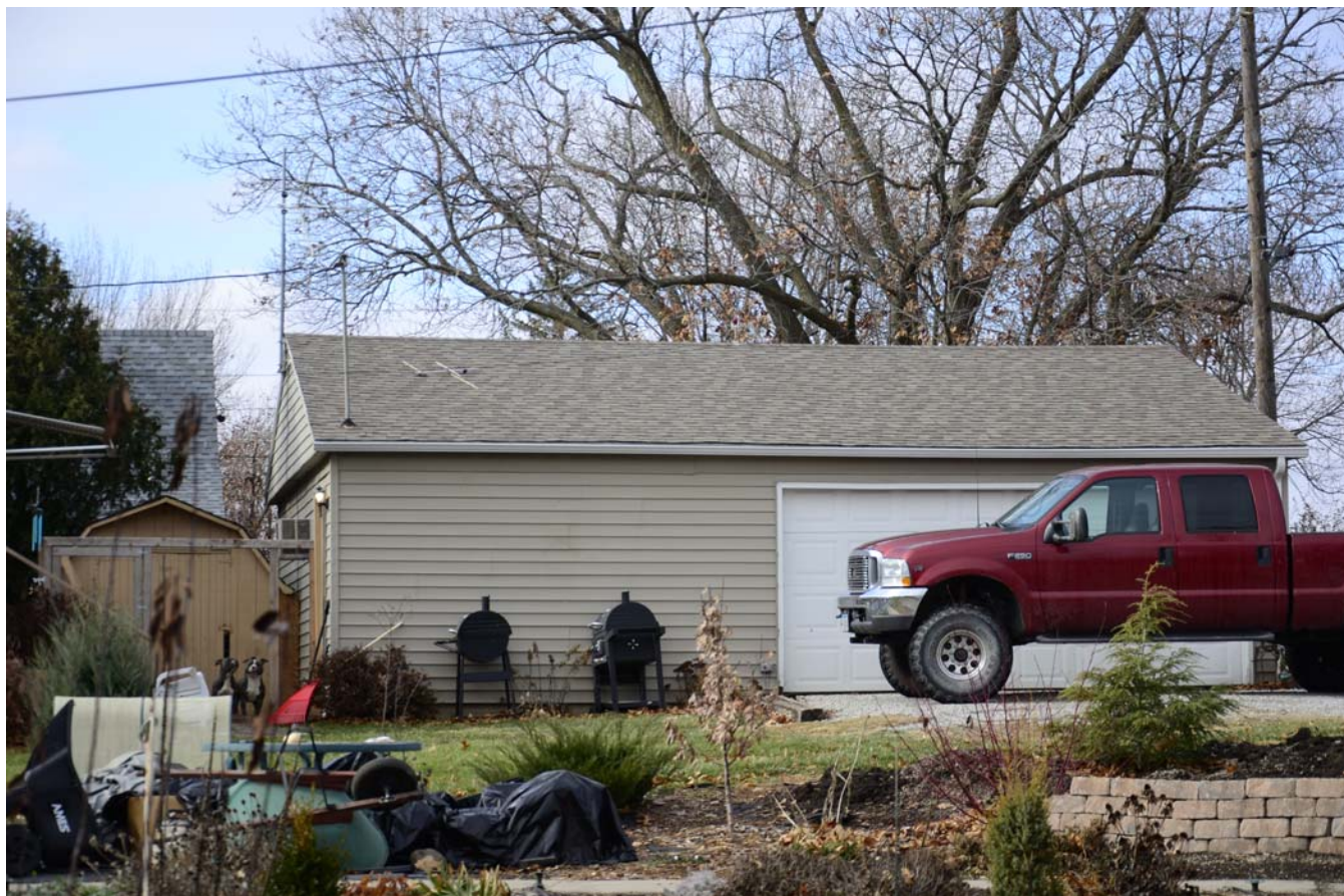
Photograph 92-00794-004 - Garage, looking west (December 2014)
