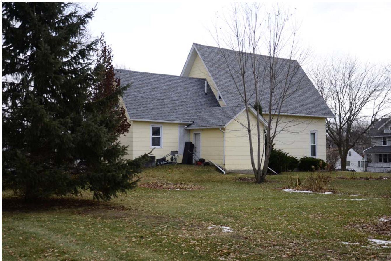
Photograph 92-00794-002 - House, looking southeast (December 2014)
