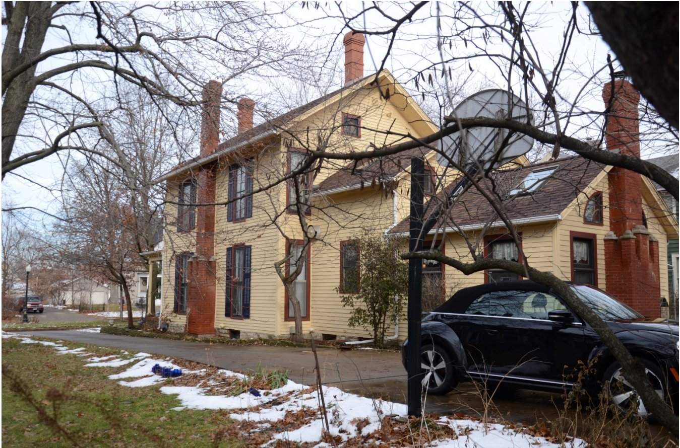
Photograph 92-00376-003 - House, looking northwest (December 2014)
