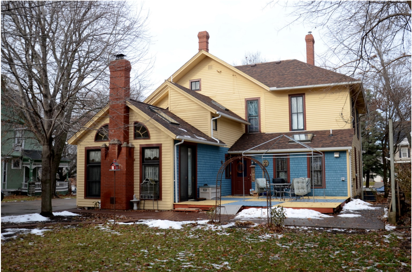
Photograph 92-00376-004 - House, looking northwest (December 2014)
