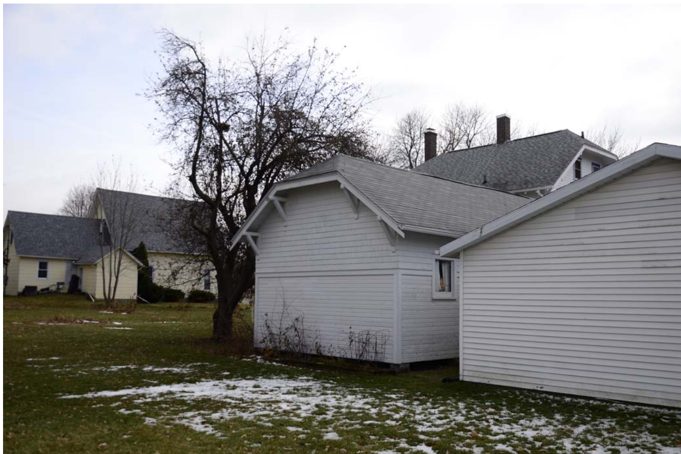
Photograph 92-00796-003 - Garage, looking southeast (December 2014)
