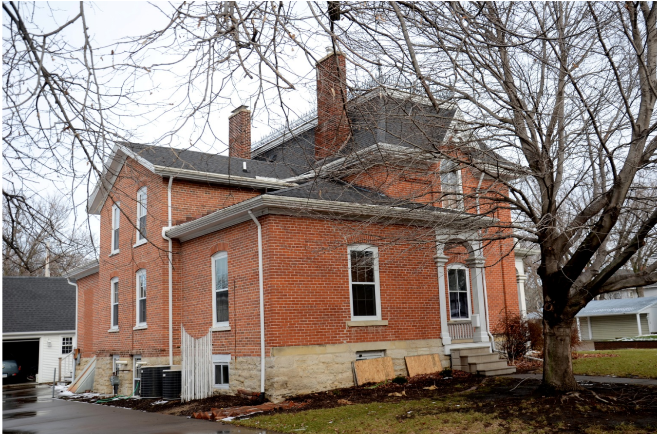
Photograph 92-00179-003 - House, looking northeast (December 2014)
