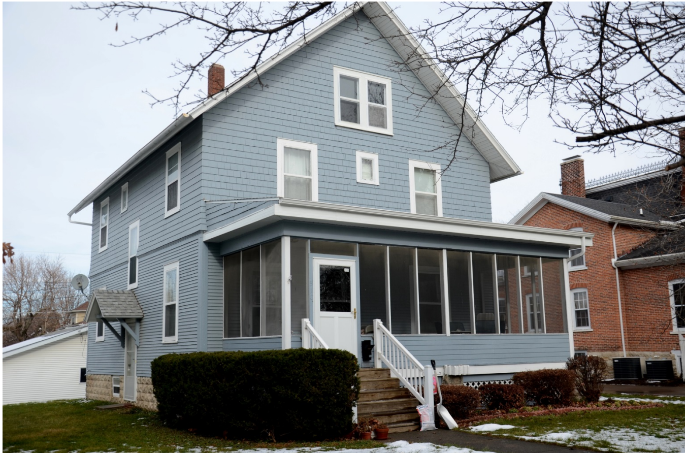
Photograph 92-00390-001 - House, looking northeast (December 2014)
