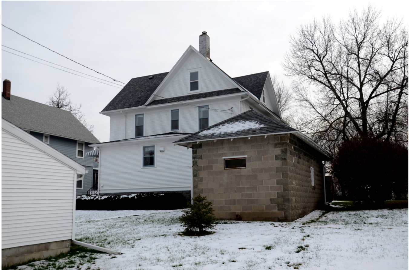
Photograph 92-00391-003 – House and garage, looking southeast (December 2014)
