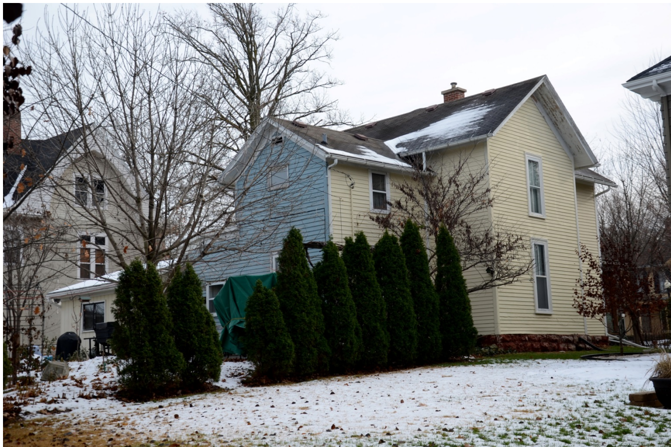
Photograph 92-00393-003 - House, looking southeast (December 2014)
