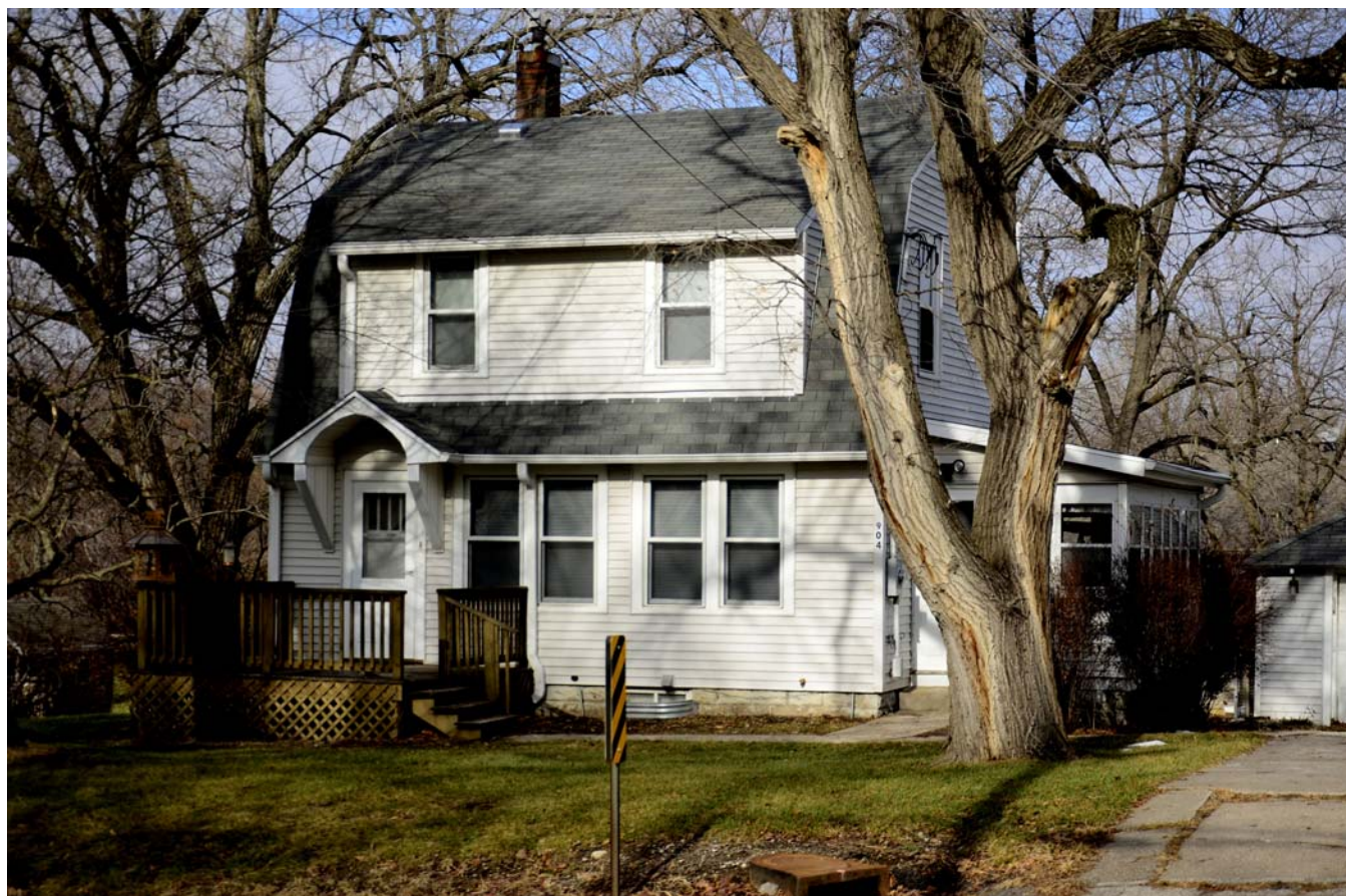
Photograph 92-00801-001 - House, looking northwest (December 2014)
