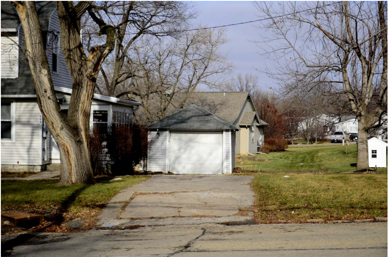
Photograph 92-00801-003 - Garage, looking north (December 2014)
