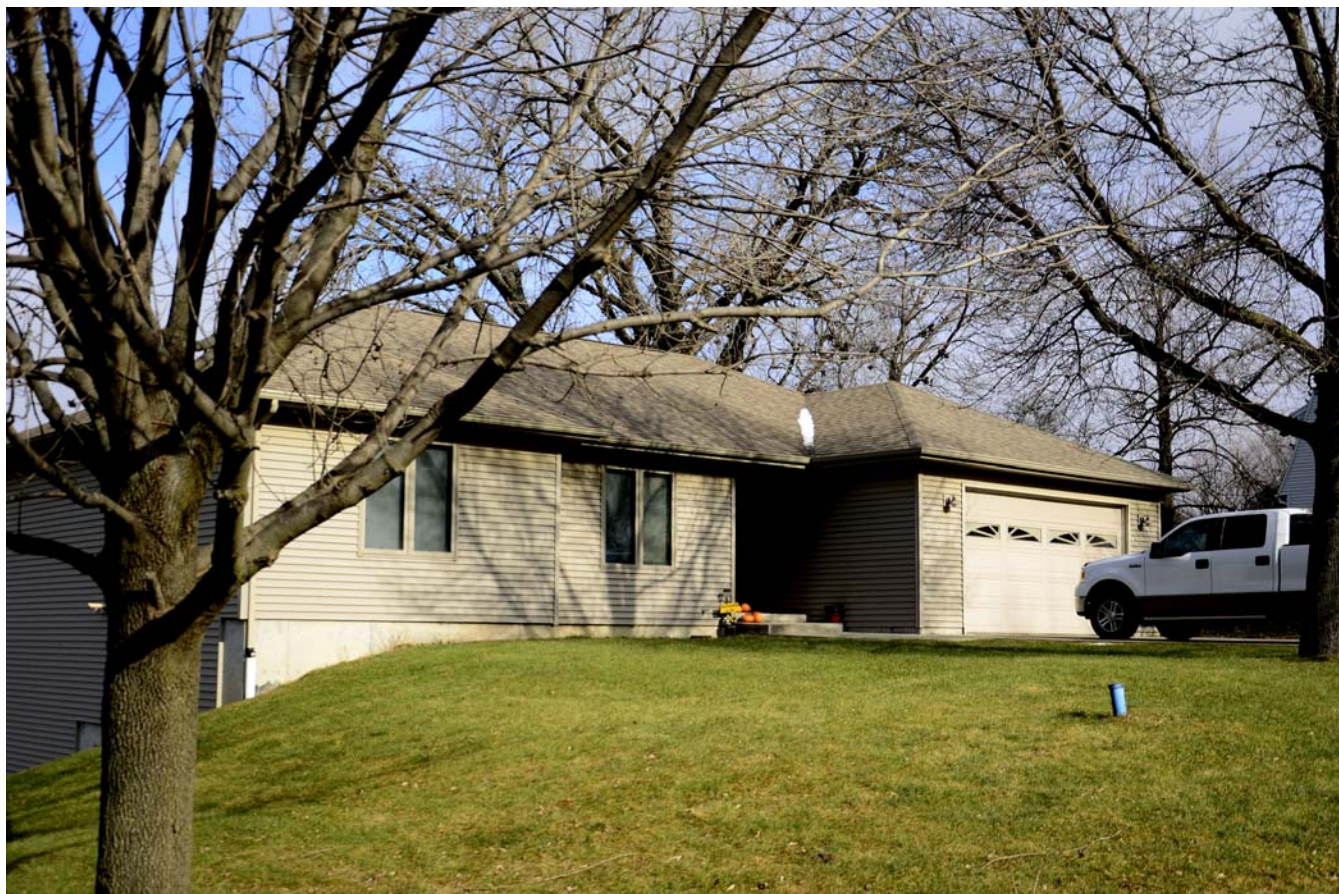
Photograph 92-00801-001 - House, looking northeast (December 2014)
