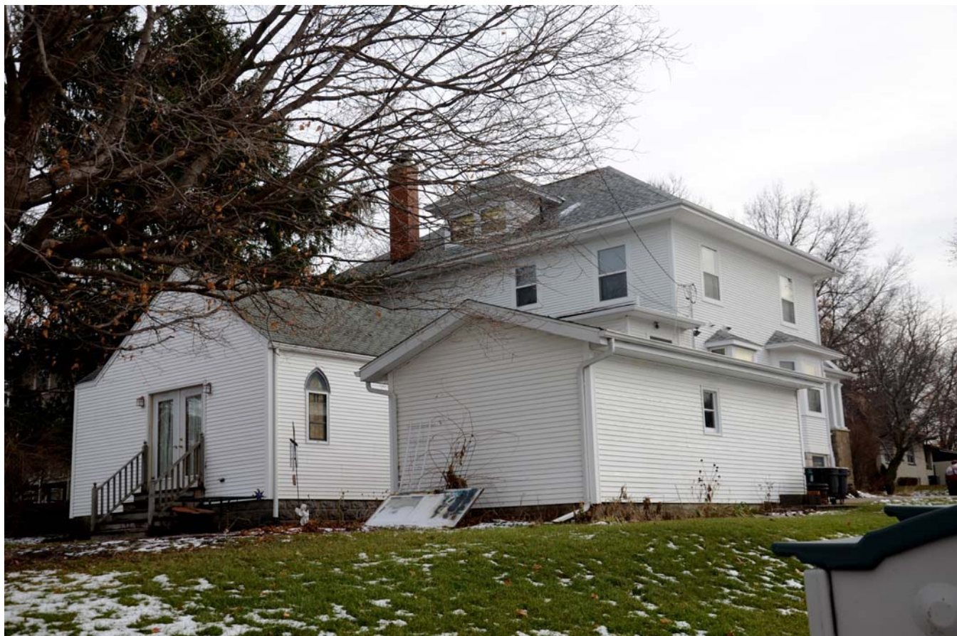
Photograph 92-00396-006 - House and garage, looking southeast (December 2014)
