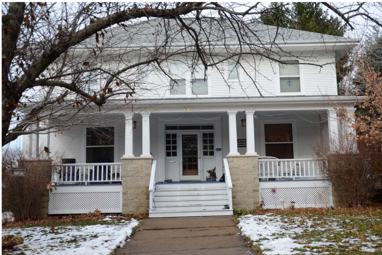
Photograph 92-00396-001 - House, looking north (December 2014)
