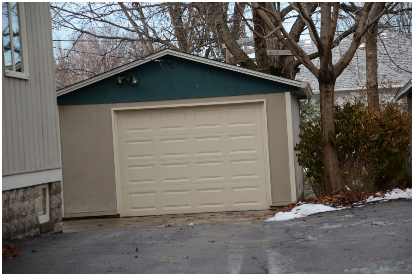
Photograph 92-00395-004 - Garage, looking north (December 2014)
