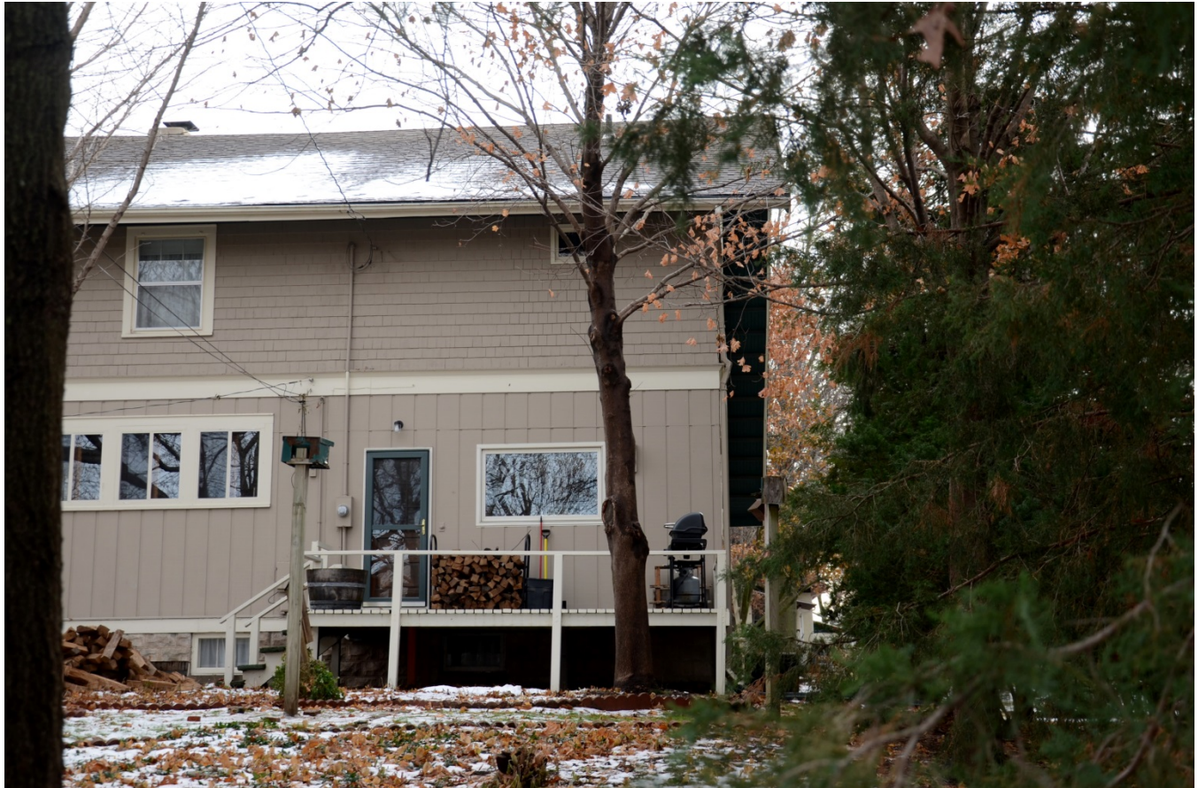
Photograph 92-00395-003 - House, looking south (December 2014)
