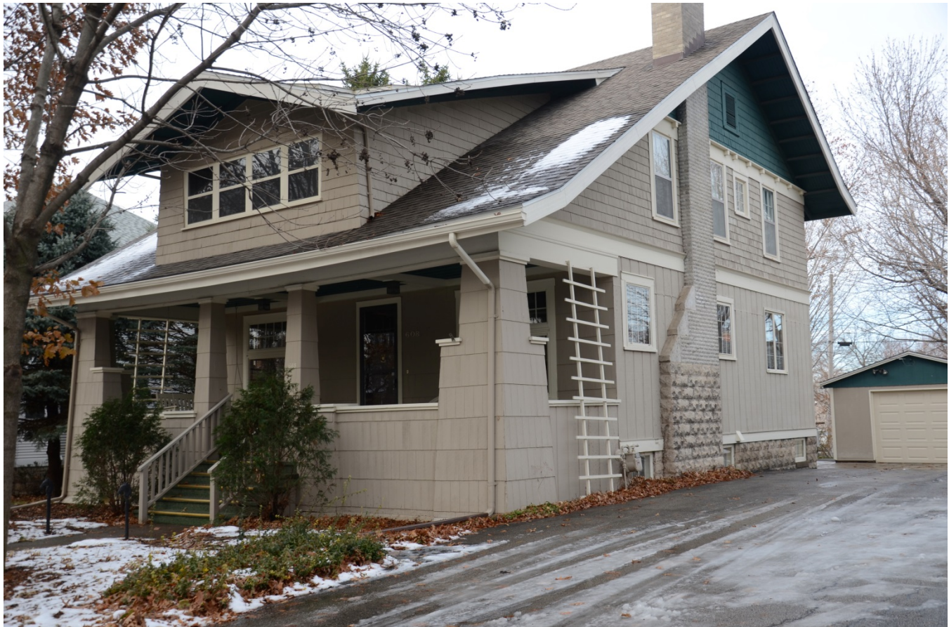
Photograph 92-00395-001 - House, looking northwest (December 2014)
