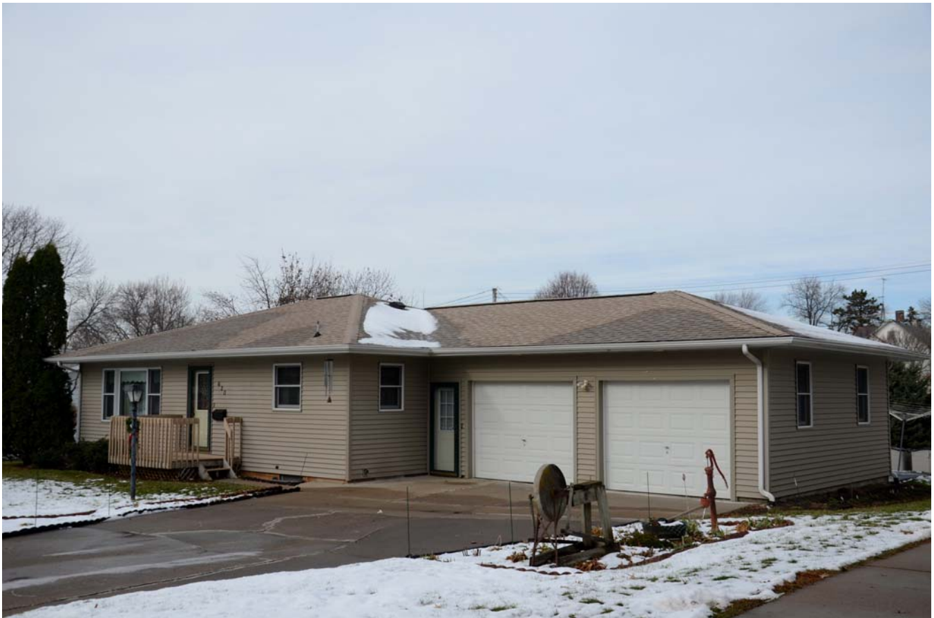
Photograph 92-00762-001 - House, looking northwest (December 2014)
