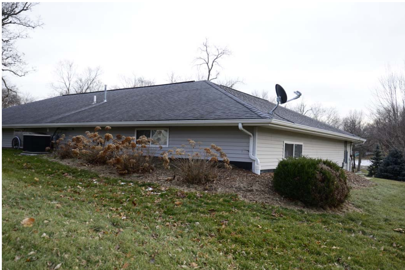
Photograph 92-00804-002 - House, looking southeast (December 2014)
