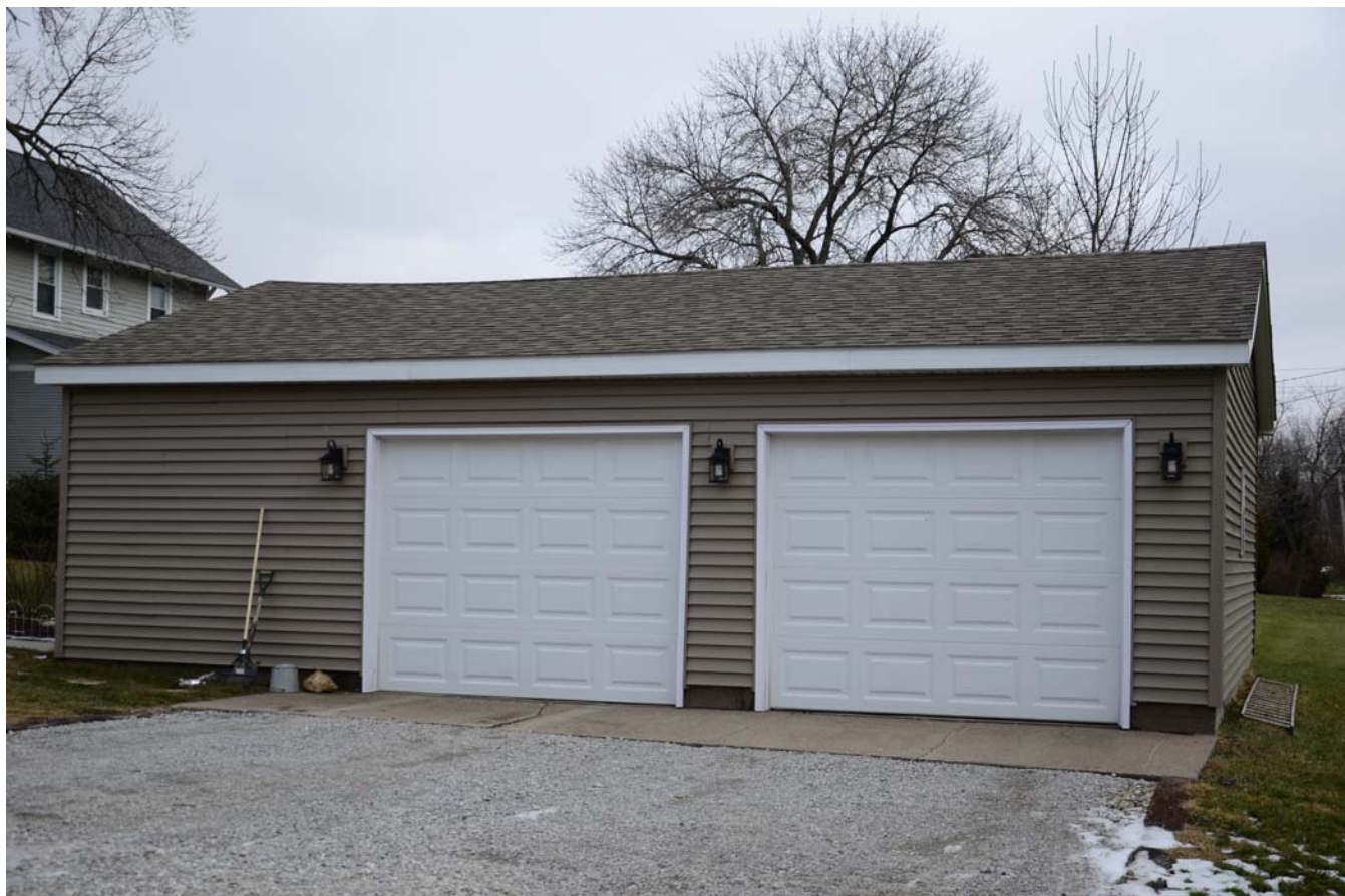
Photograph 92-00789-004 - Garage, looking east (December 2014)
