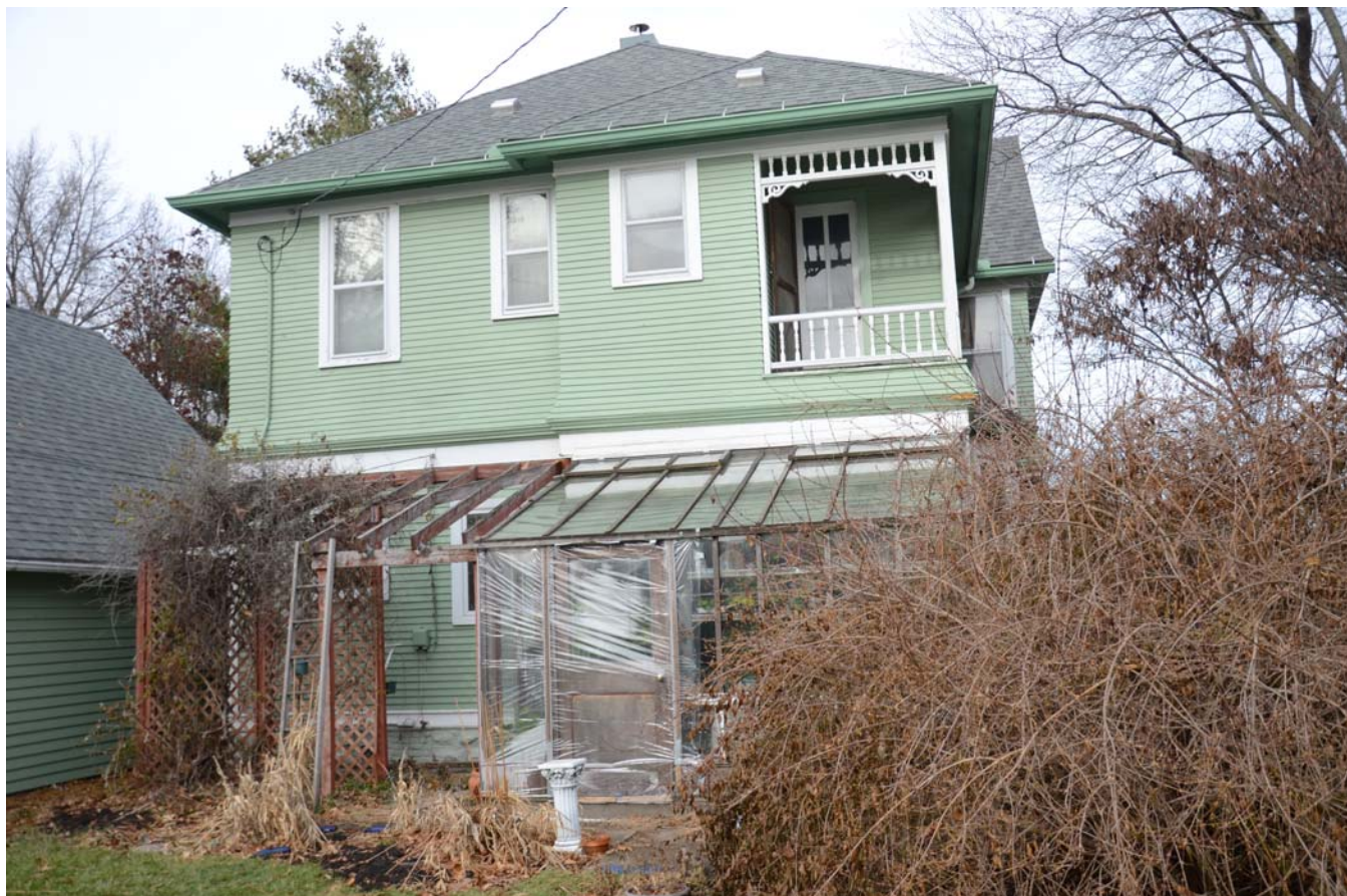
Photograph 92-00180-004 - House, looking north (December 2014)
