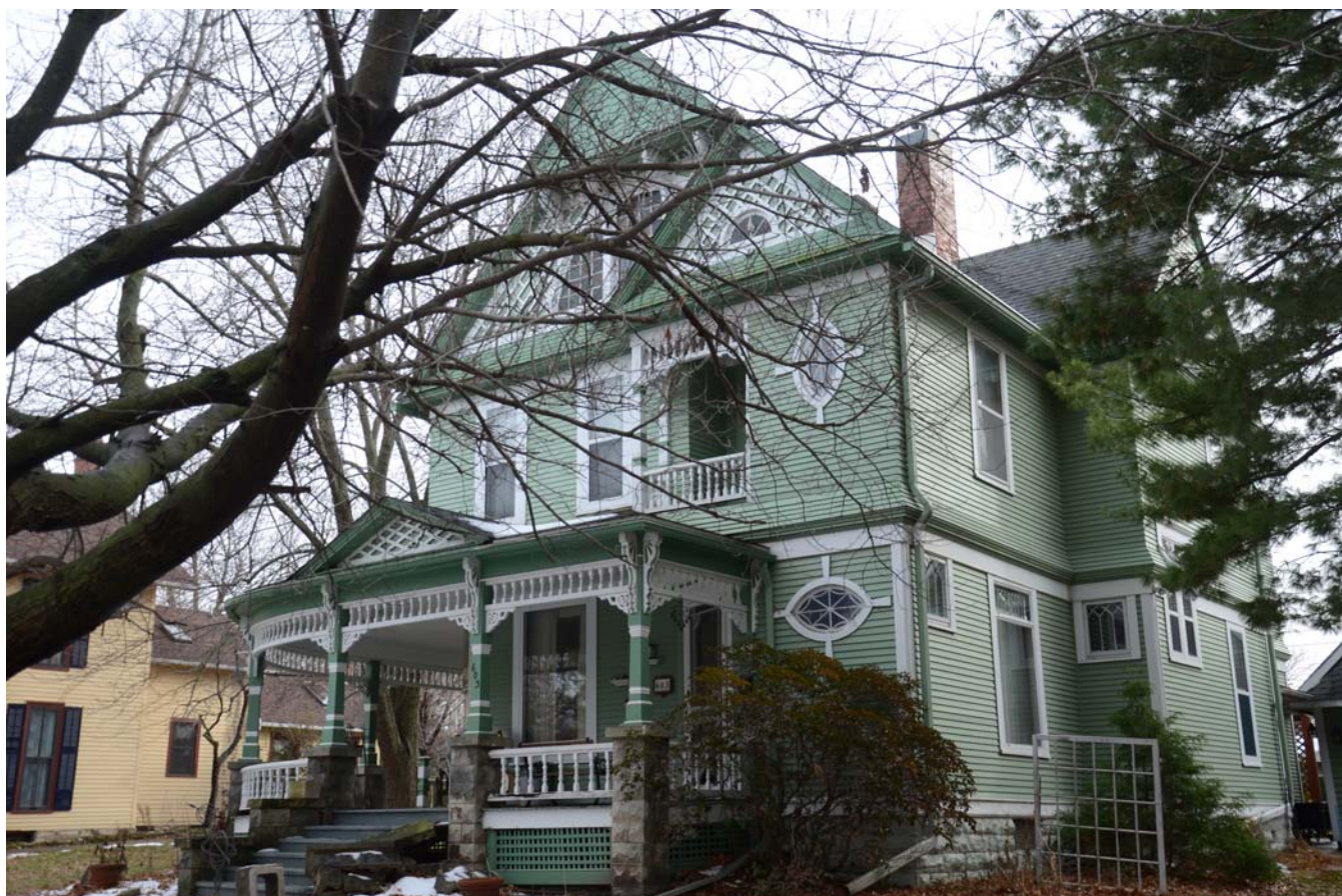
Photograph 92-00180-001 - House, looking southeast (December 2014)
