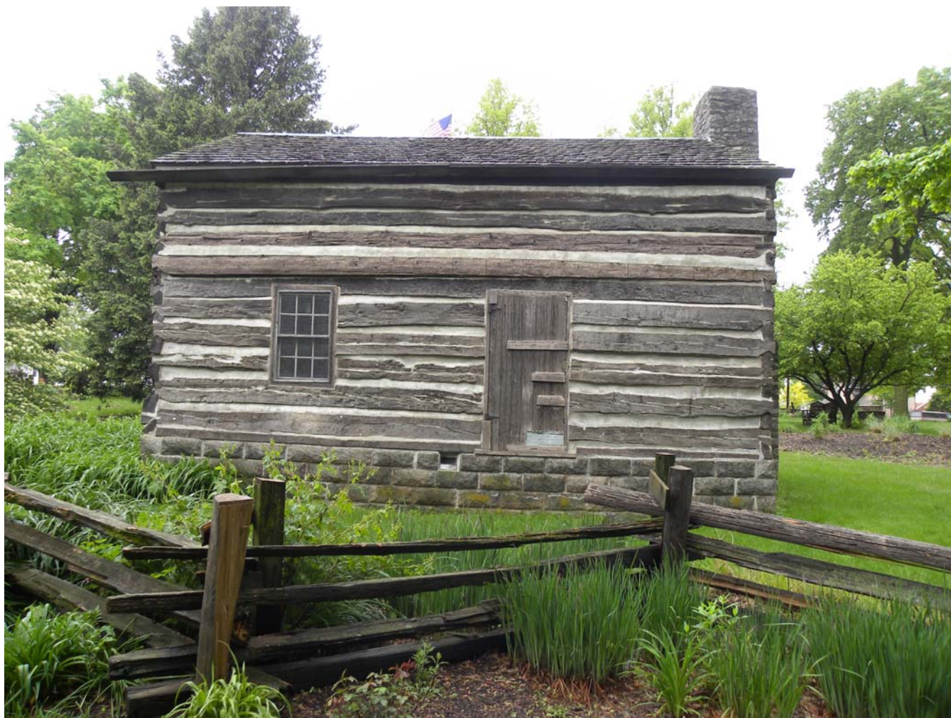
Photograph 92-00160-002 - Log House, looking south (July 2015)
