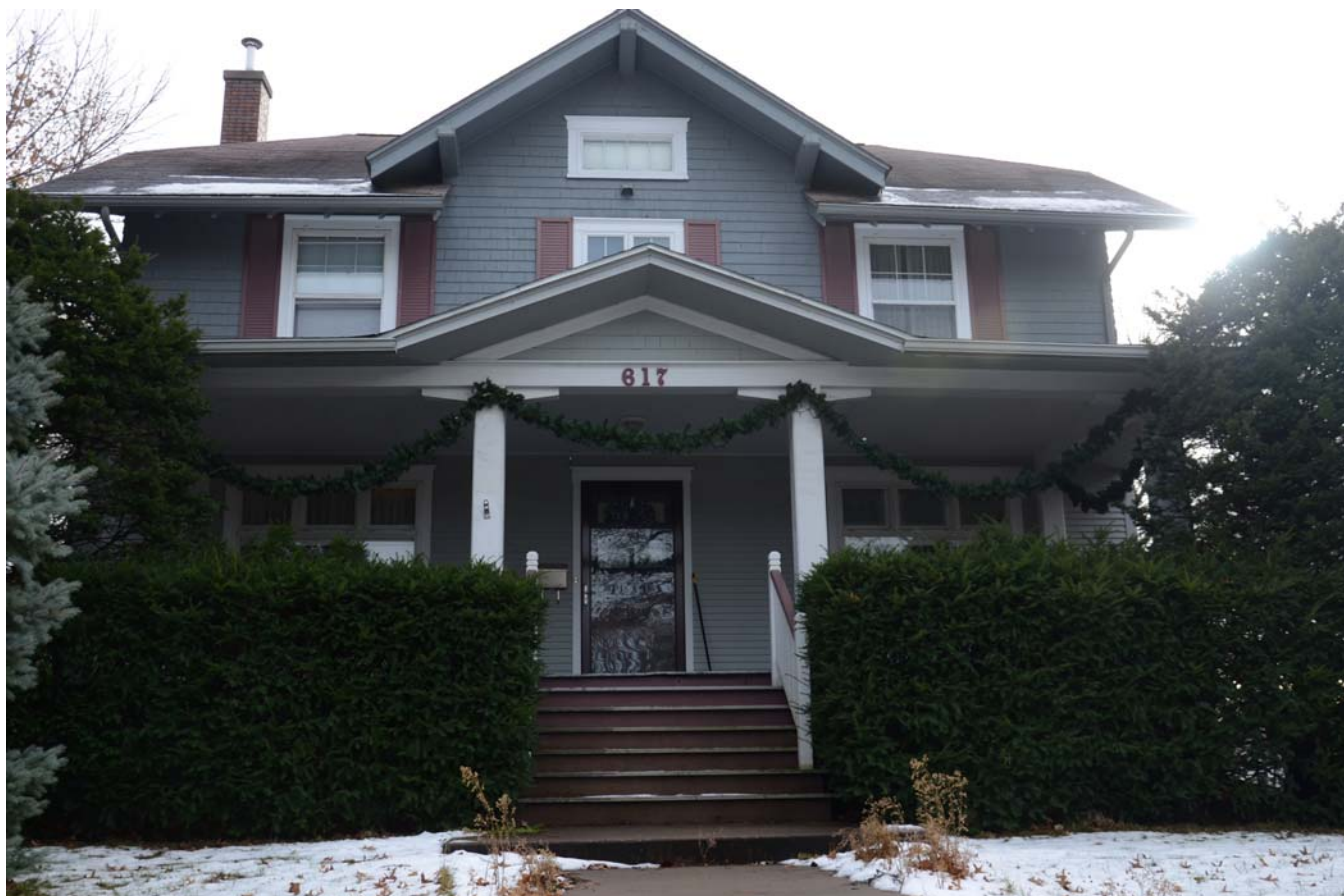
Photograph 92-00379-001 - House, looking south (December 2014)
