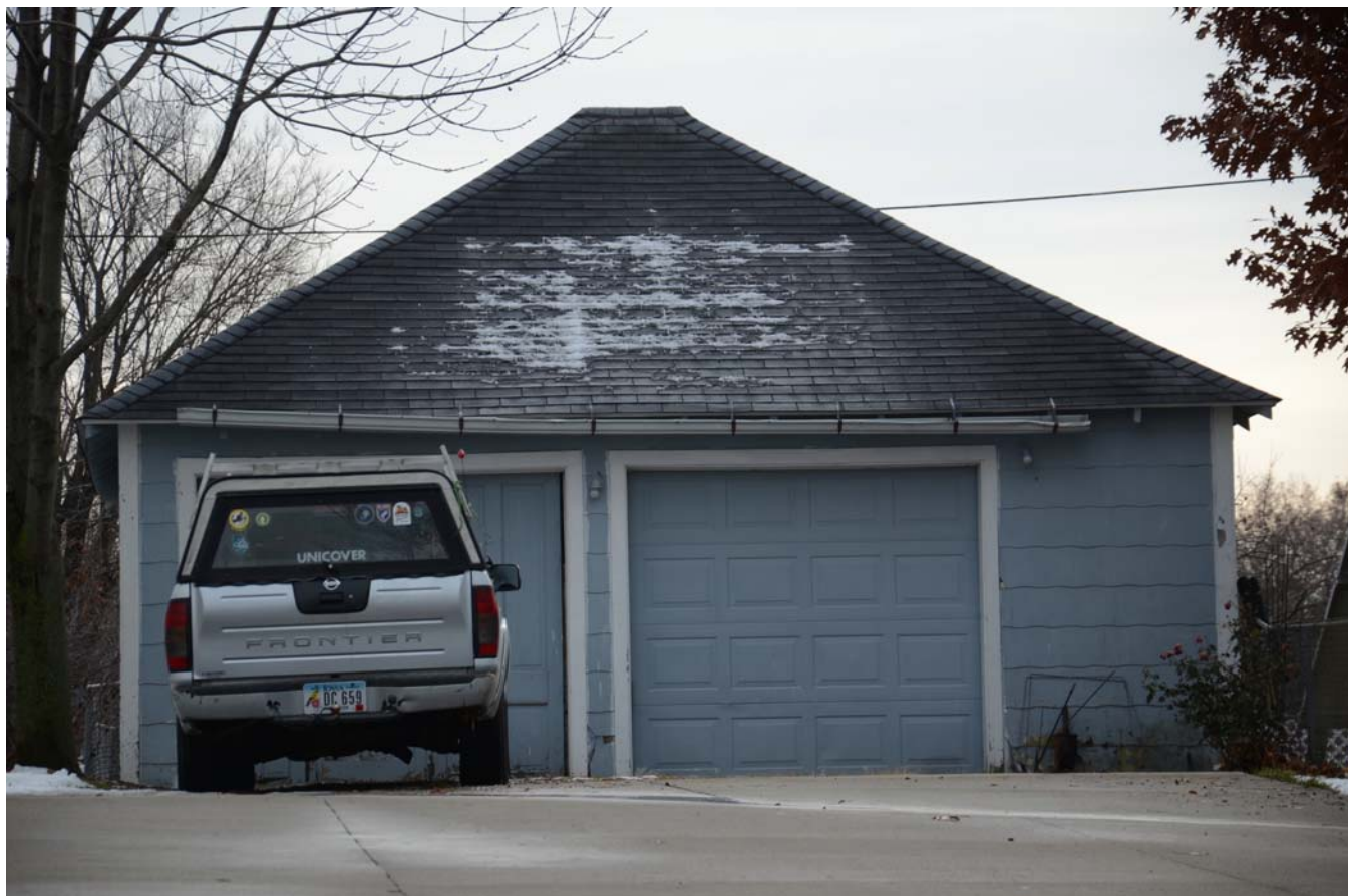
Photograph 92-00381-004 - Garage, looking south (December 2014)
