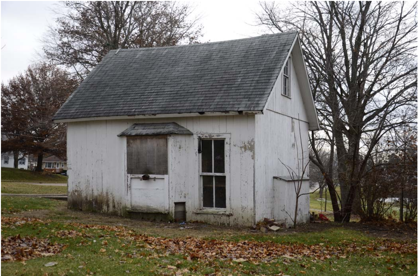
Photograph 92-00435-005 - Garage, looking southeast (December 2014)
