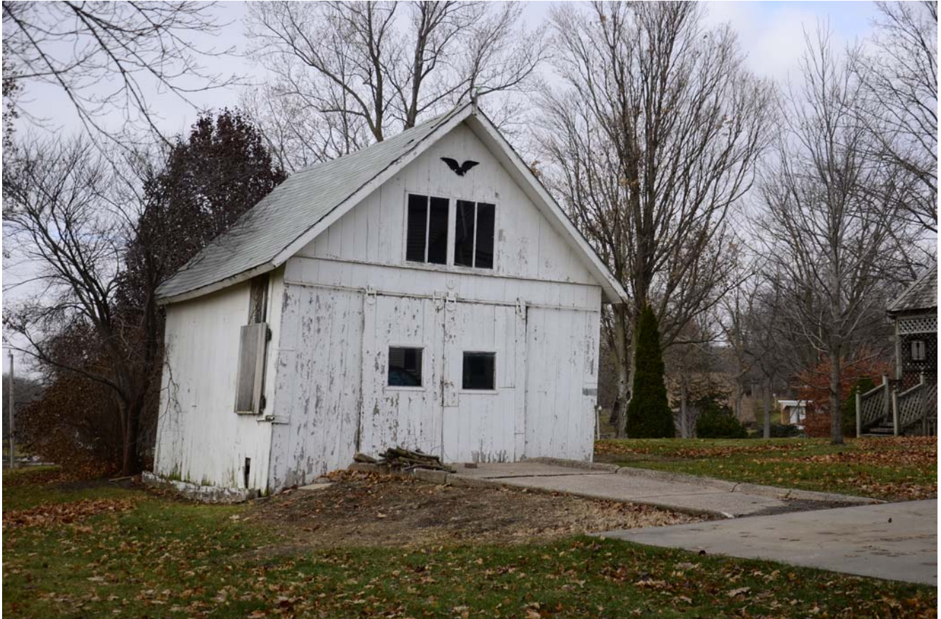
Photograph 92-00431-004 - Garage, looking northwest (December 2014)
