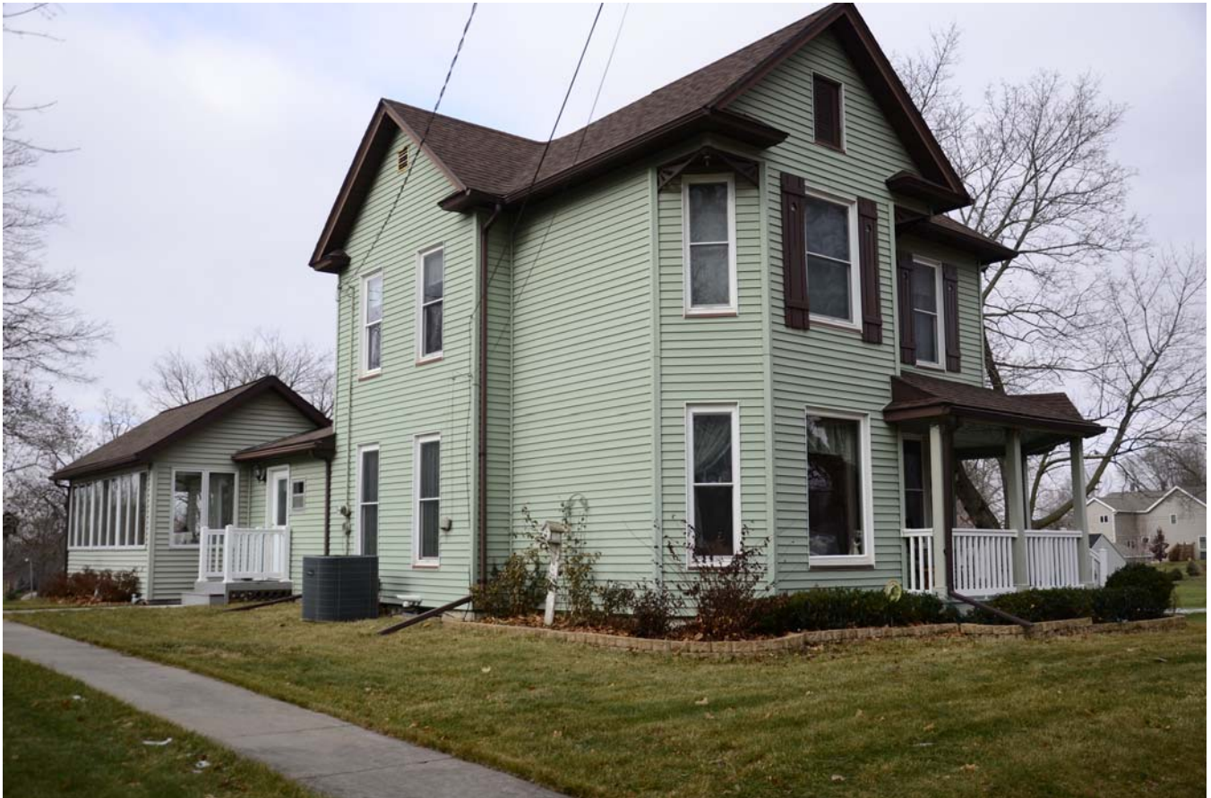
Photograph 92-00765-002 - House, looking northwest (December 2014)
