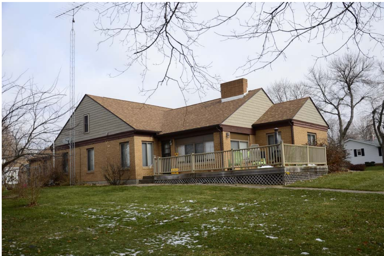
Photograph 92-00766-002 - House, looking northeast (December 2014)
