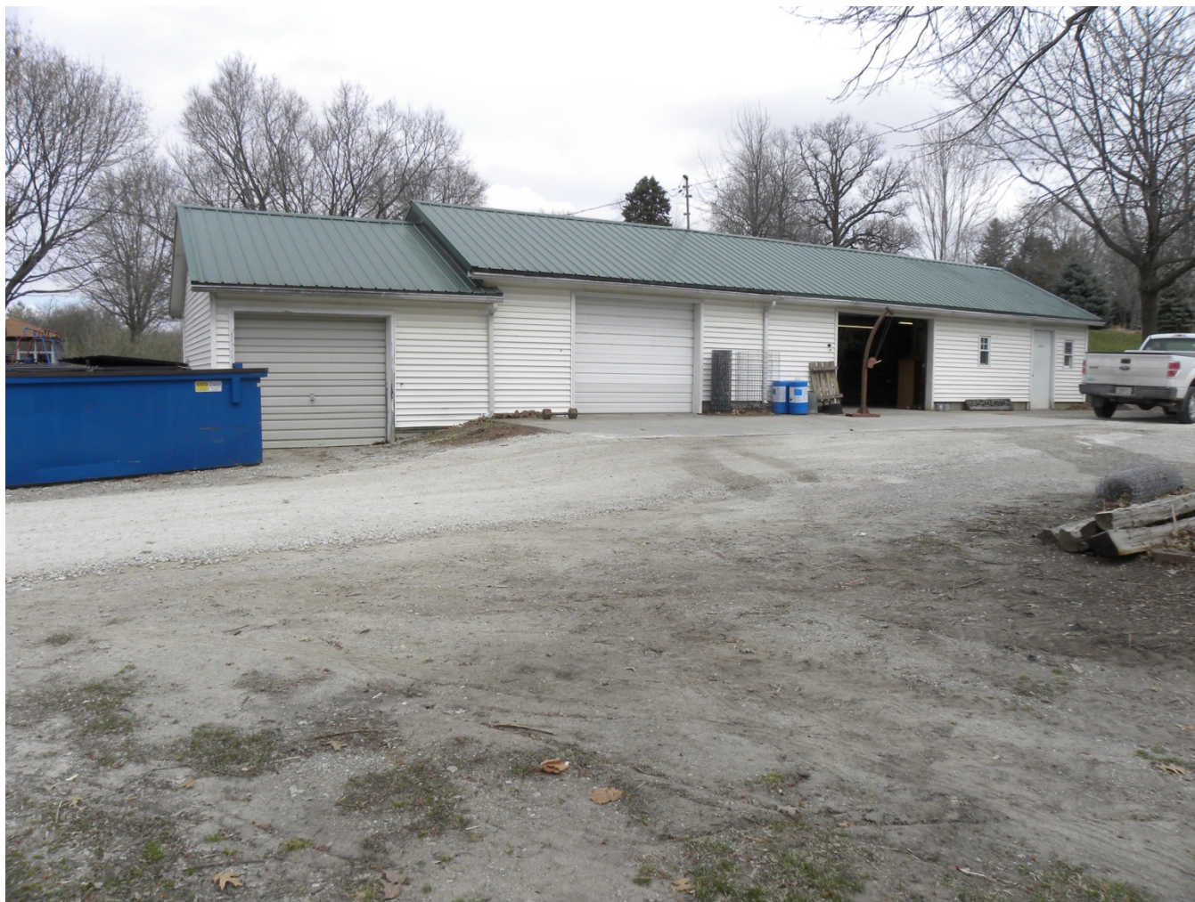
Photograph 92-00805-027 – Maintenance building (B1) at east end of Section 5, looking north (December 2014)
