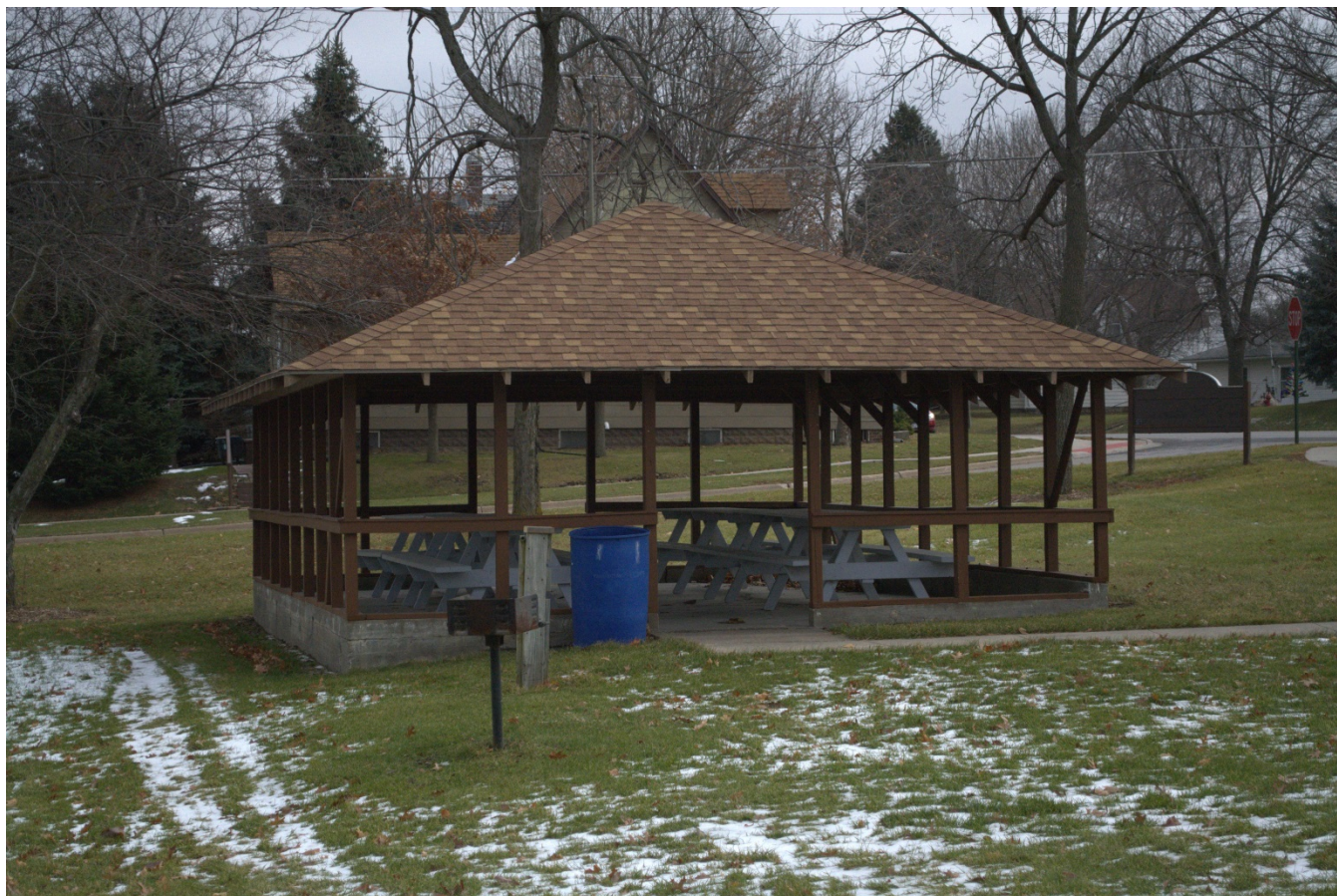
Photograph 92-00805-005 - Shelter 2 in Section 2, looking east (December 2014)
