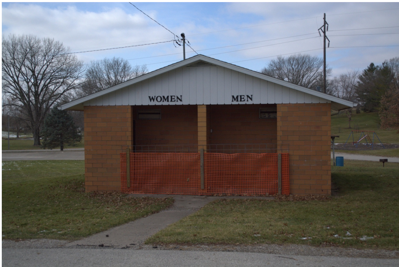
Photograph 92-00805-029 – Restrooms (R2) in middle part of Section 5, looking west (December 2014)
