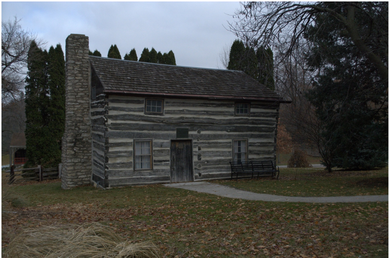
Photograph 92-00805-008 - Alexander Young Log House, looking northeast (December 2014)
