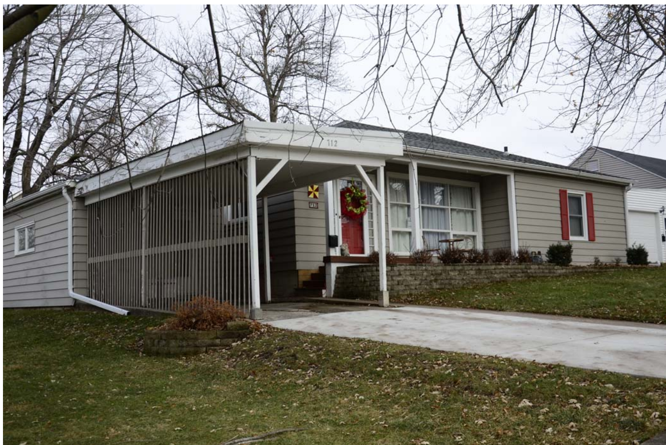
Photograph 92-00768-001 - House, looking northeast (December 2014)
