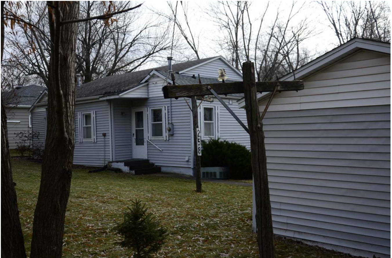
Photograph 92-00769-003 - House, looking southeast (December 2014)
