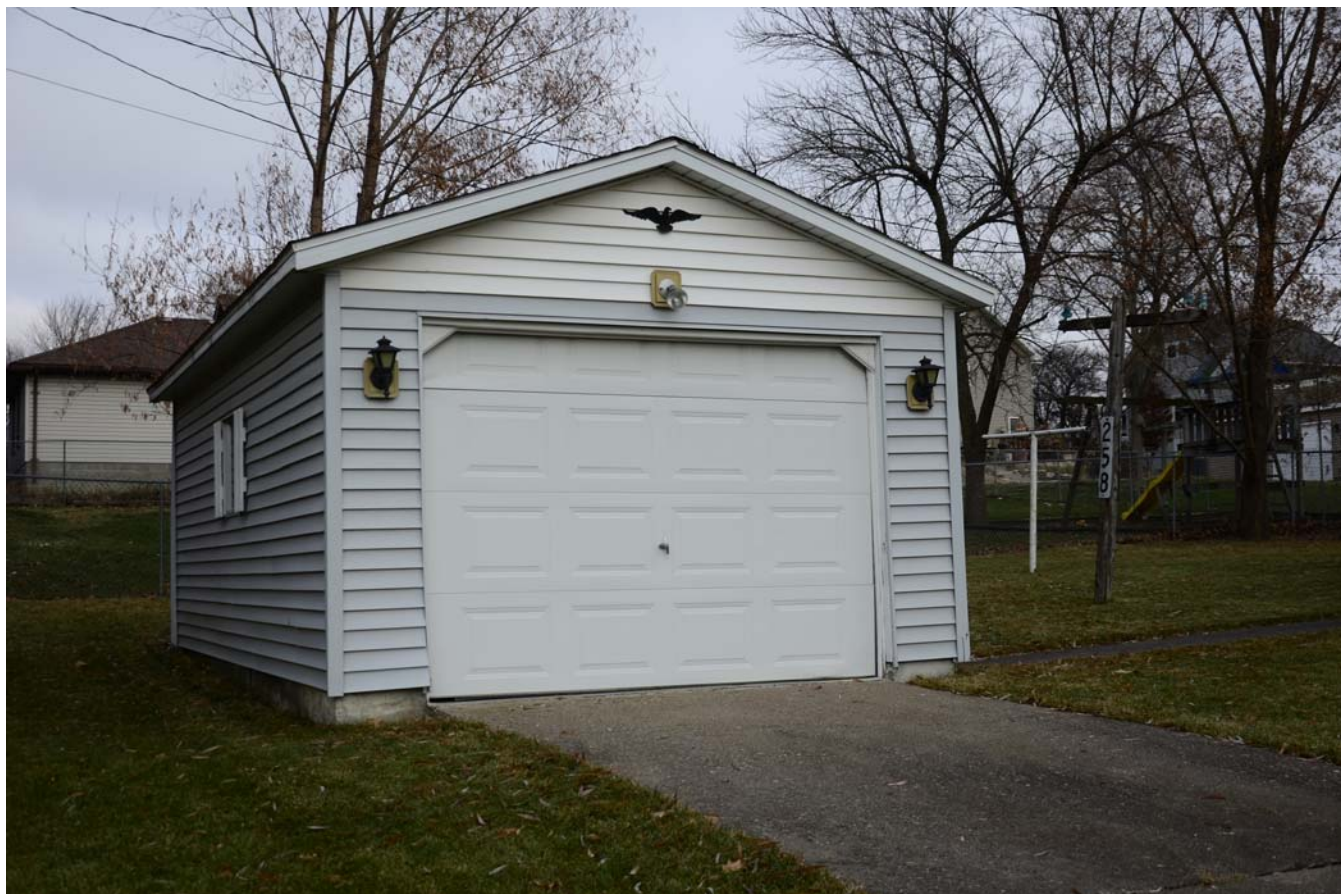
Photograph 92-00769-004 - Garage, looking northeast (December 2014)
