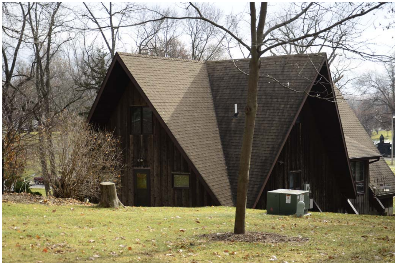
Photograph 92-00771-002 - House, looking southeast (December 2014)
