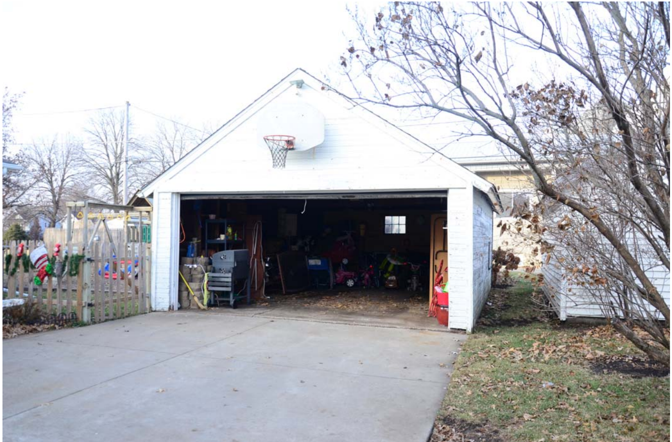
Photograph 92-00411-006 - Garage, looking northwest (December 2014)
