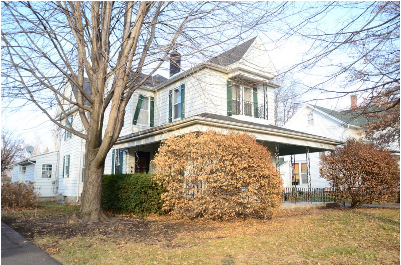
Photograph 92-00411-002 - House, looking northeast (December 2014)
