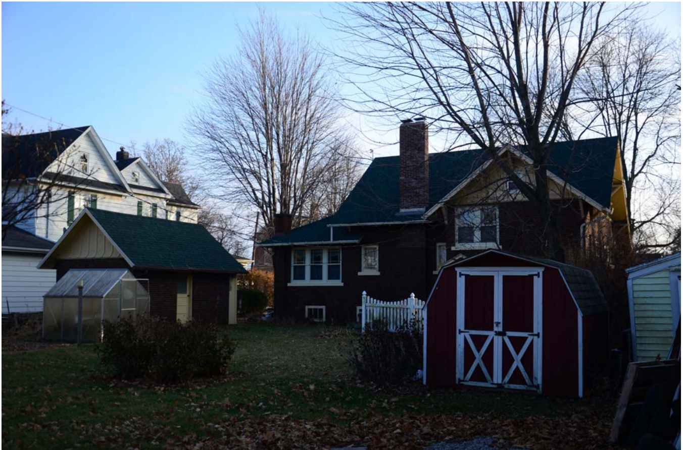
Photograph 92-00412-003 - House, looking northeast (December 2014)
