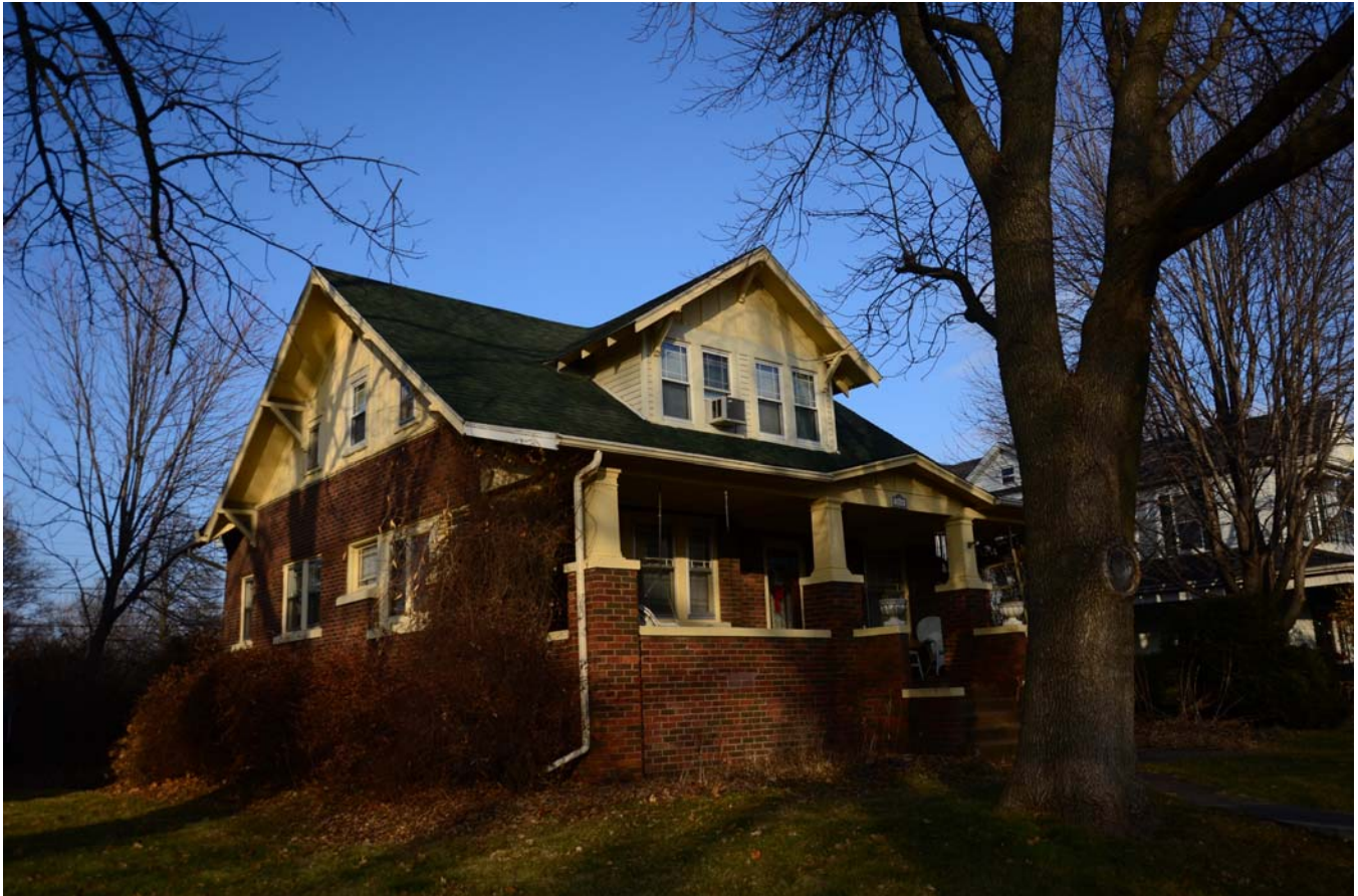
Photograph 92-00412-001 - House, looking northeast (December 2014)
