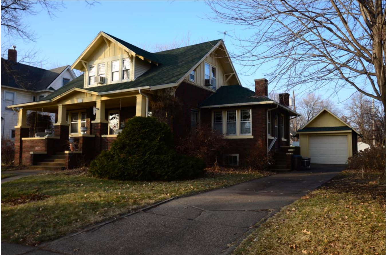
Photograph 92-00412-002 - House, looking northeast (December 2014)
