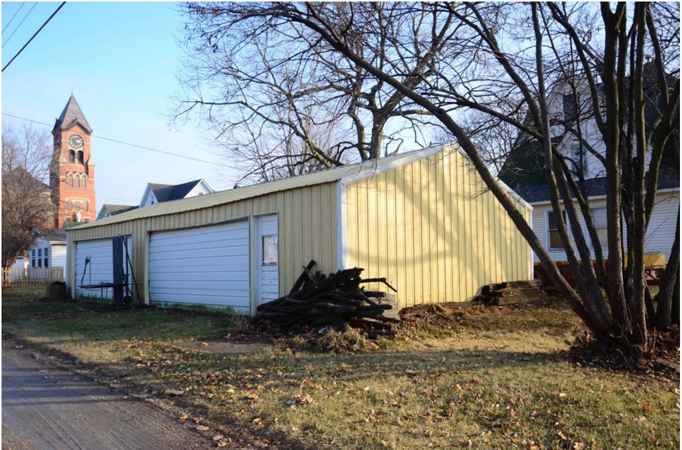
Photograph 92-00413-004 - Garage, looking southeast (December 2014)
