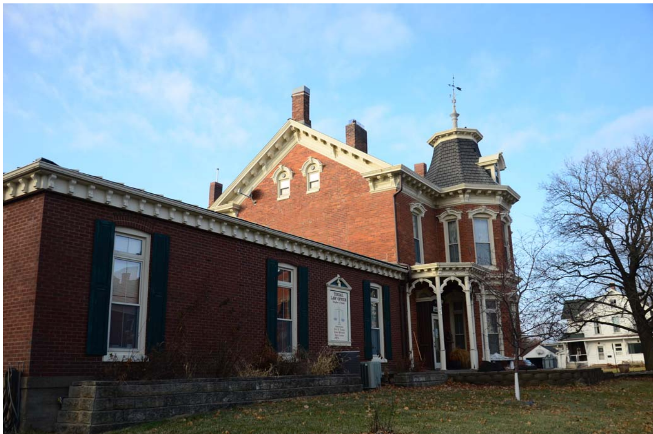
Photograph 92-00397-003 - House, looking northwest (December 2014)
