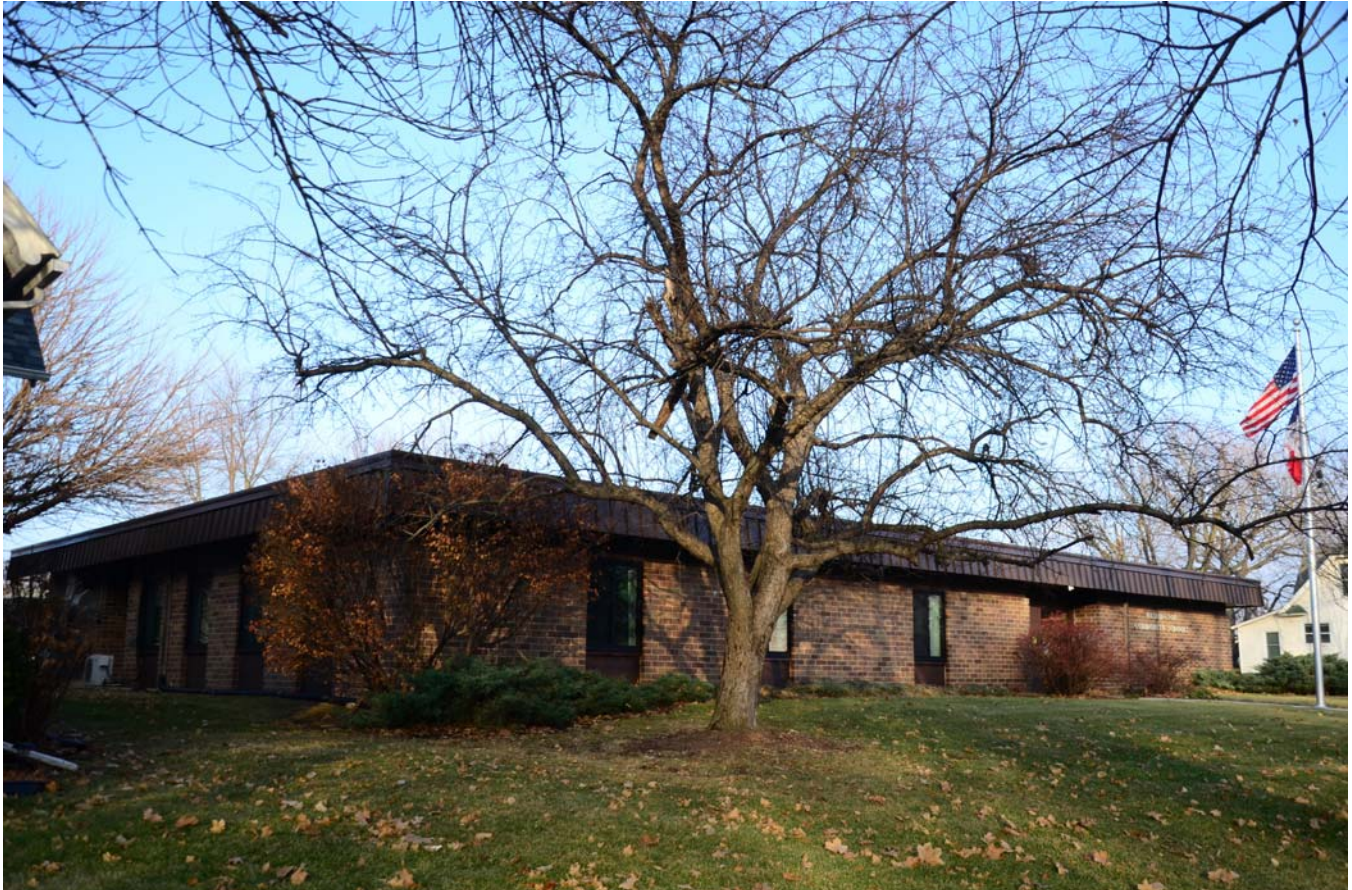
Photograph 92-00774-002 - Building, looking northeast (December 2014)
