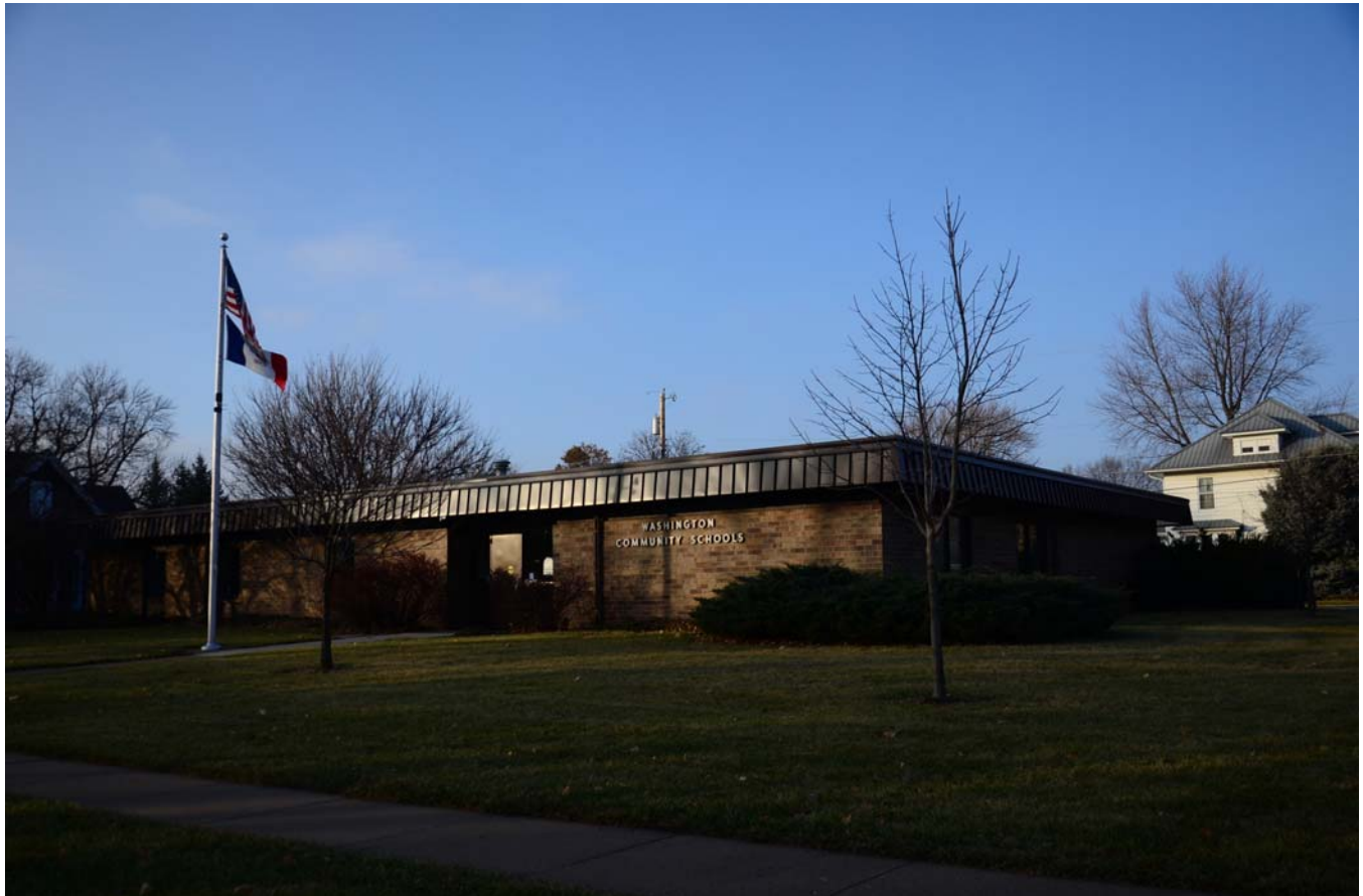
Photograph 92-00774-001 - Building, looking northwest (December 2014)
