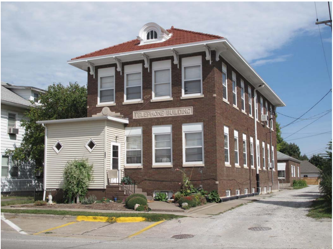
Photograph 92-00661-001 - West and south elevations, looking northeast (McCarley, September 20, 2011).
