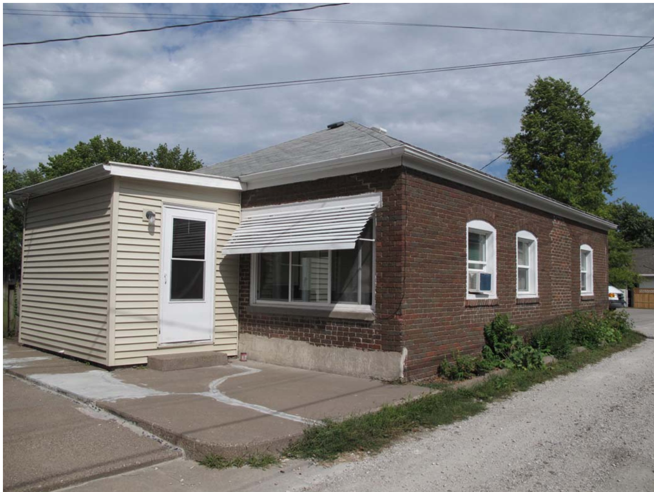
Photograph 92-00661-007 - West and south elevations of converted garage, looking northeast (McCarley, September 20, 2011).
