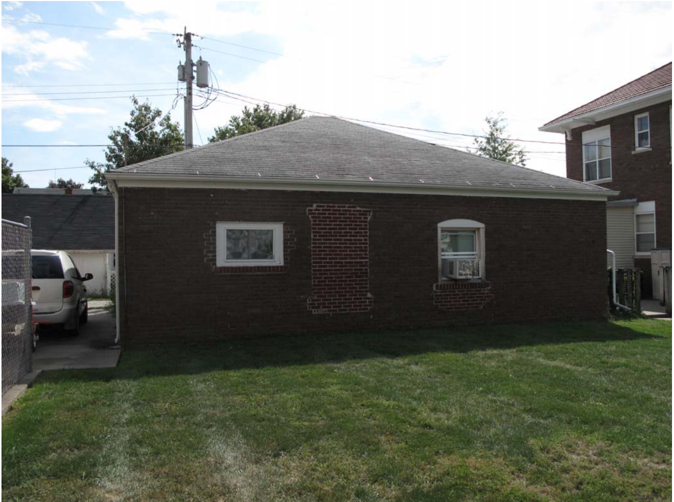
Photograph 92-00661-009 - North elevation of converted garage, looking south (McCarley, September 20, 2011).
