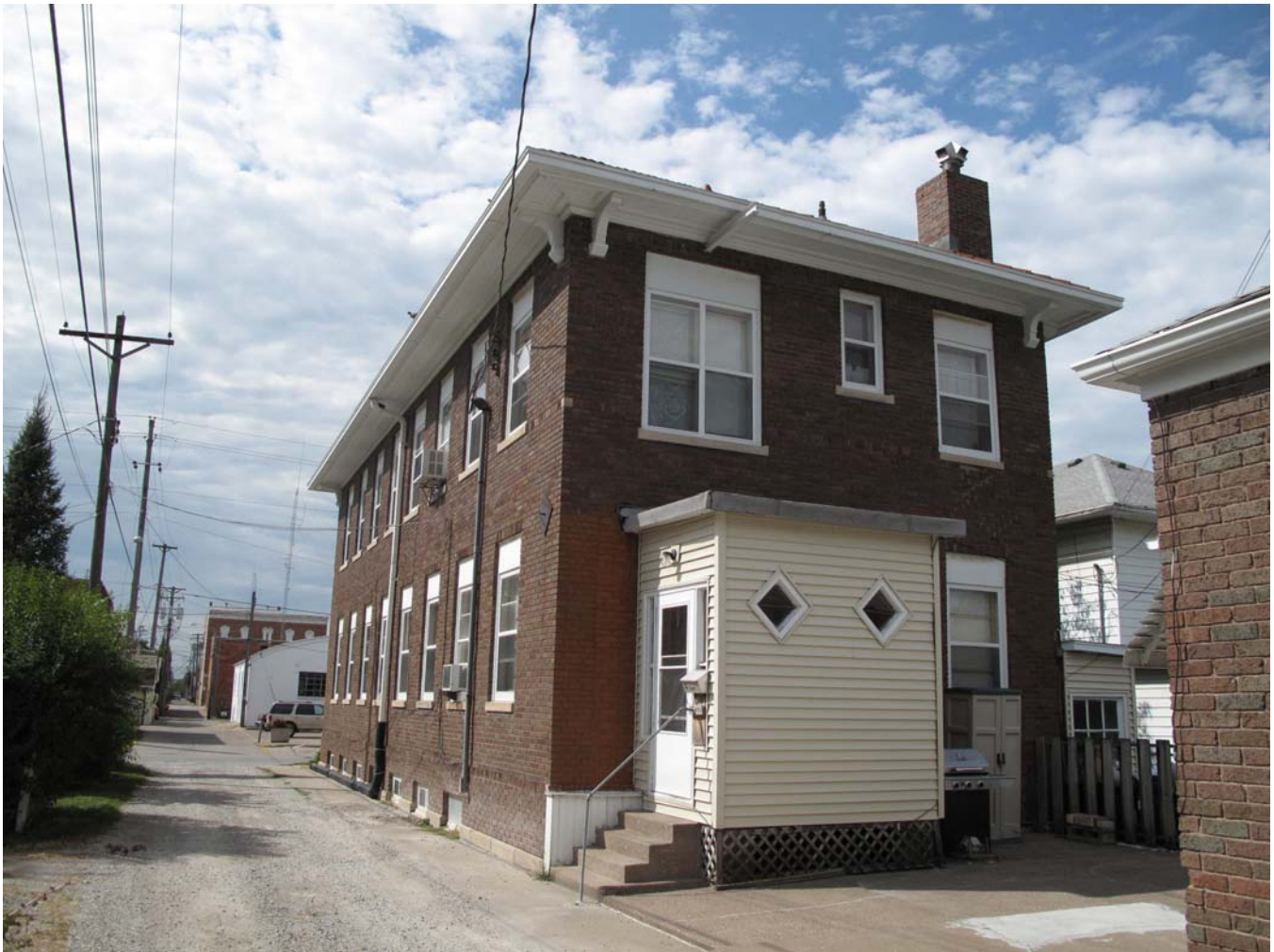
Photograph 92-00661-005 - South and east elevations, looking northwest (McCarley, September 20, 2011).
