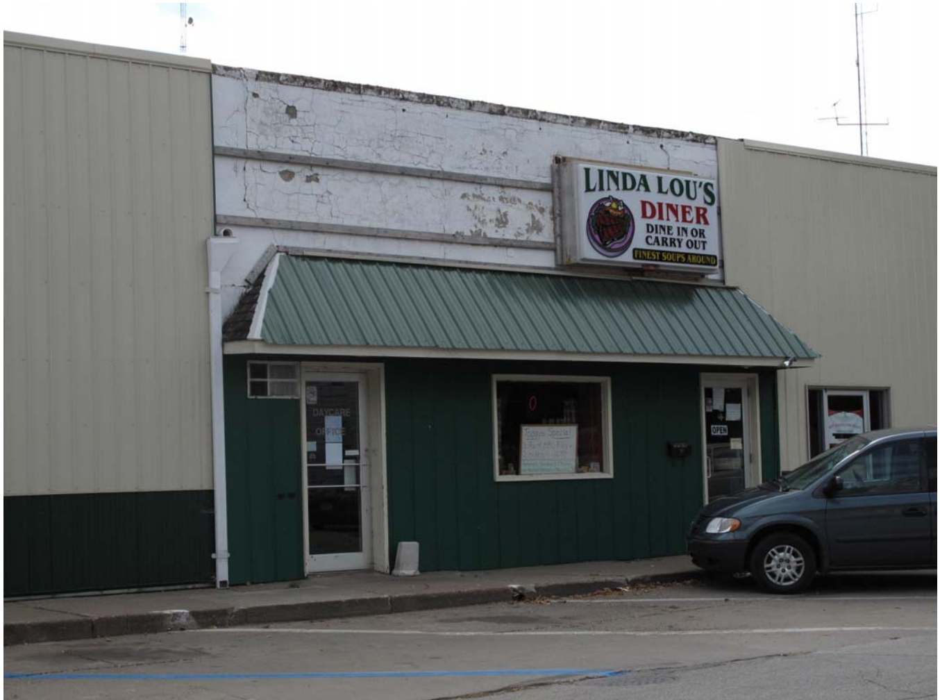
Photograph 92-00578-002 - North elevation of 117 section, looking southwest (McCarley, September 20, 2011)
