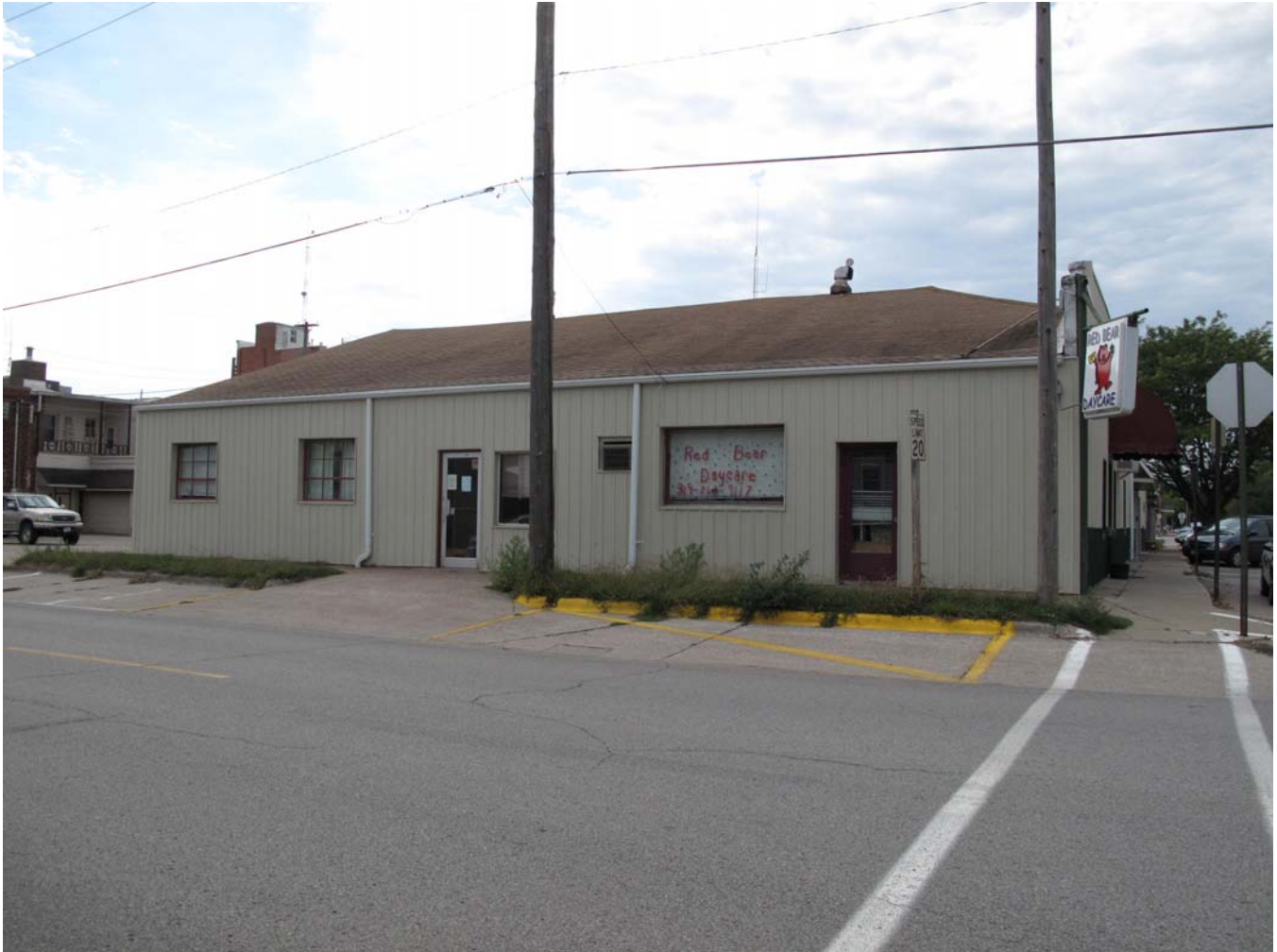
Photograph 92-00578-003 - East elevation, looking west (McCarley, September 20, 2011)
