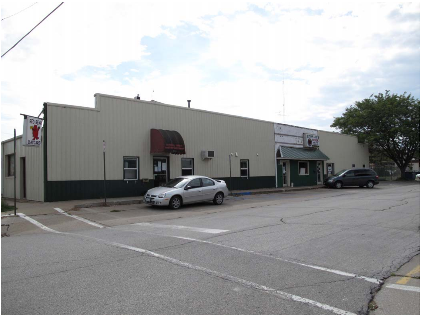
Photograph 92-00578-001 - North elevation, looking southwest (McCarley, September 20, 2011)
