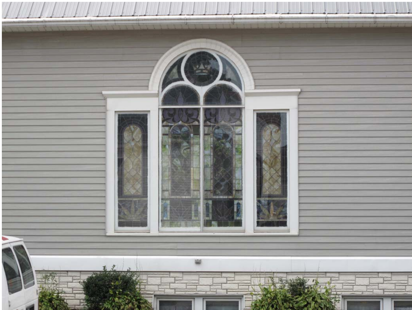
Photograph 92-00579-004 - Detail of window on east elevation, looking west (McCarley, September 20, 2011)
