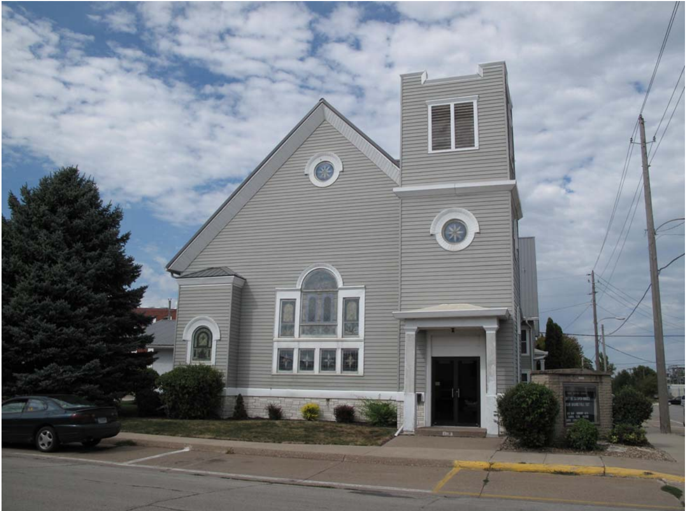
Photograph 92-00579-002 - South elevation, looking north (McCarley, September 20, 2011)
