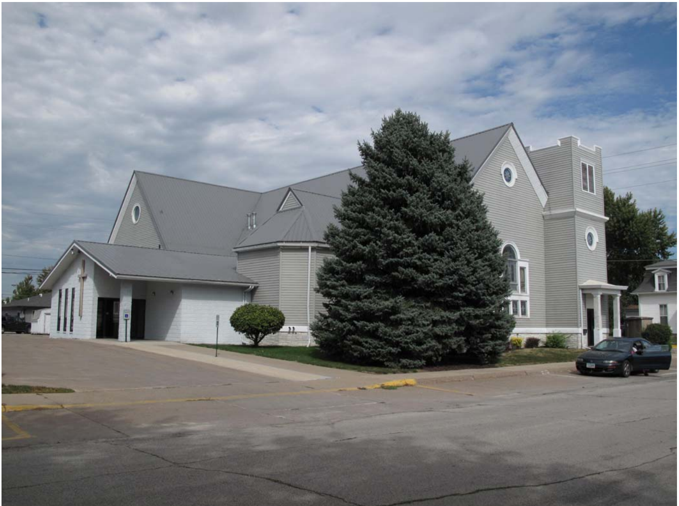
Photograph 92-00579-005 - West and south elevations, looking northeast (McCarley, September 20, 2011)
