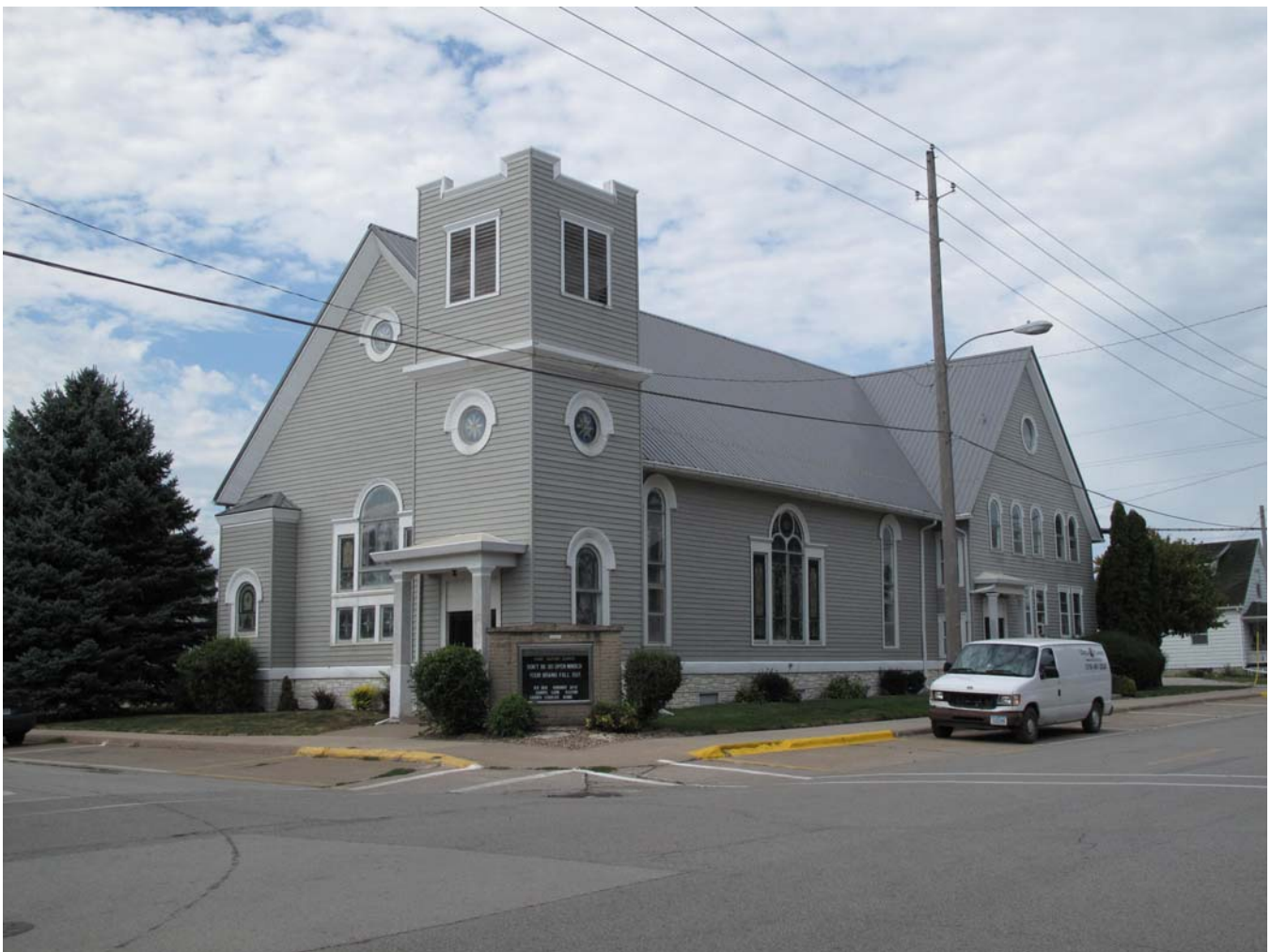
Photograph 92-00579-001 - South and east elevations, looking northwest (McCarley, September 20, 2011)
