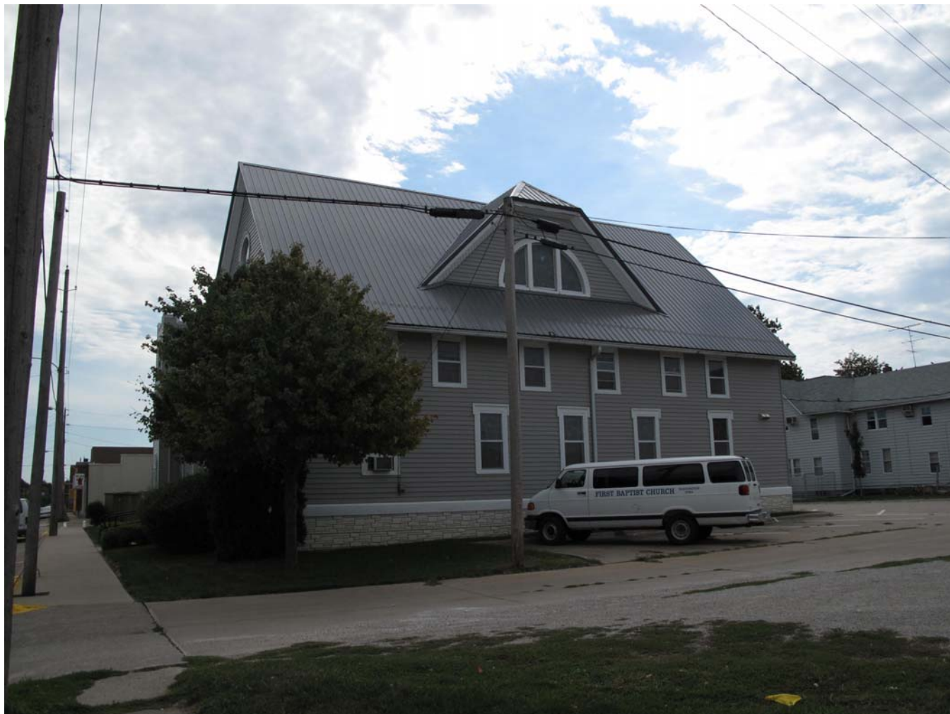
Photograph 92-00579-006 - North elevation, looking south (McCarley, September 20, 2011)
