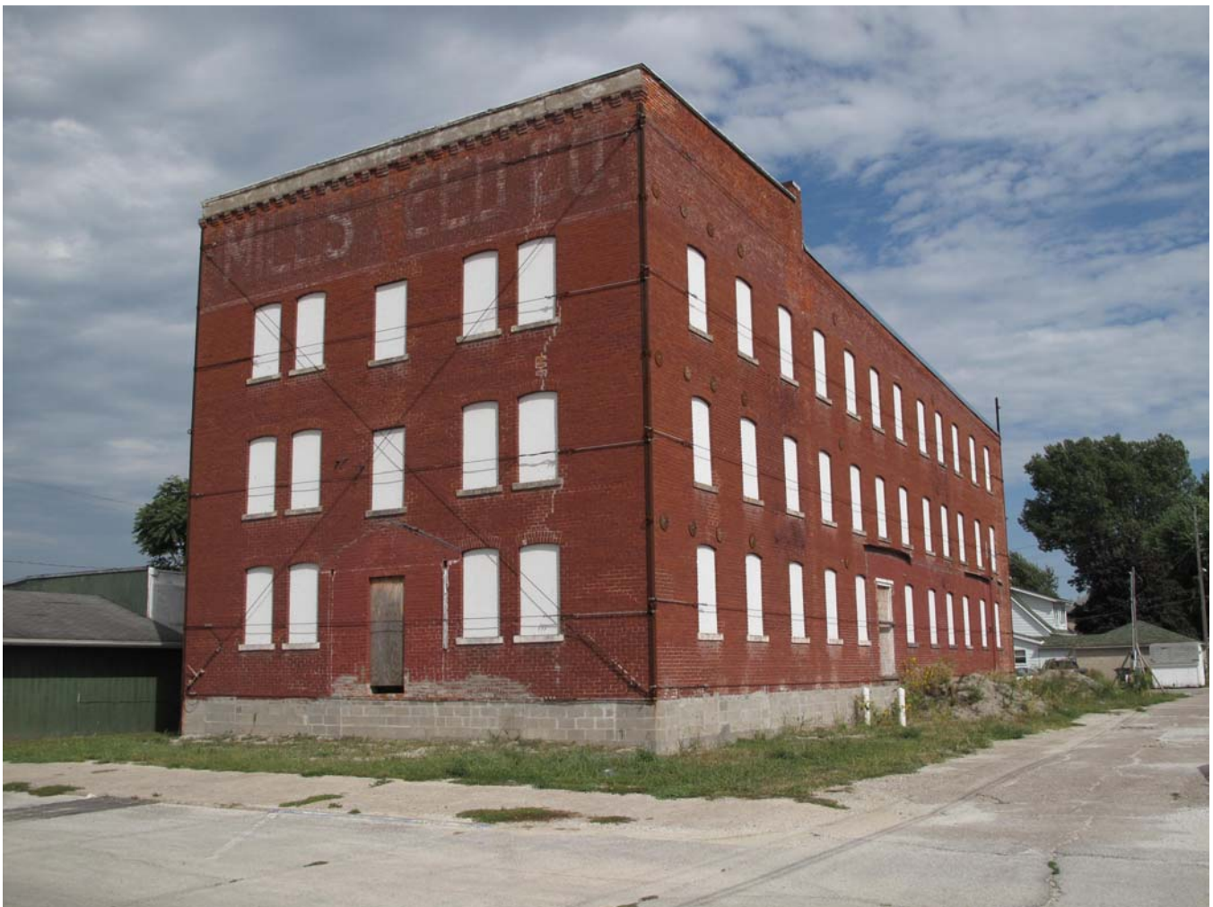
Photograph 92-00471-001 - West and south elevations, looking northeast (McCarley, September 20, 2011)
