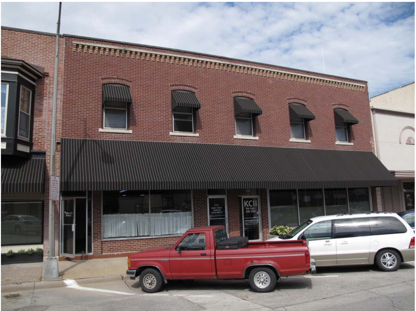
Photograph 92-00533-001 - South elevation, looking northeast (September 20, 2011).
