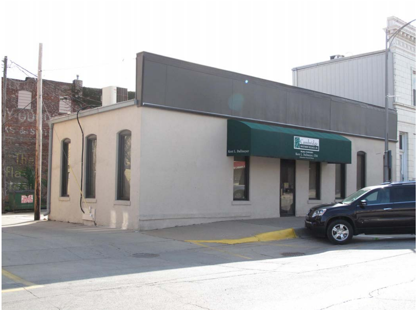
Photograph 92-00508-004 - East and north elevations of rear section, looking southwest (McCarley, September 20, 2011)
