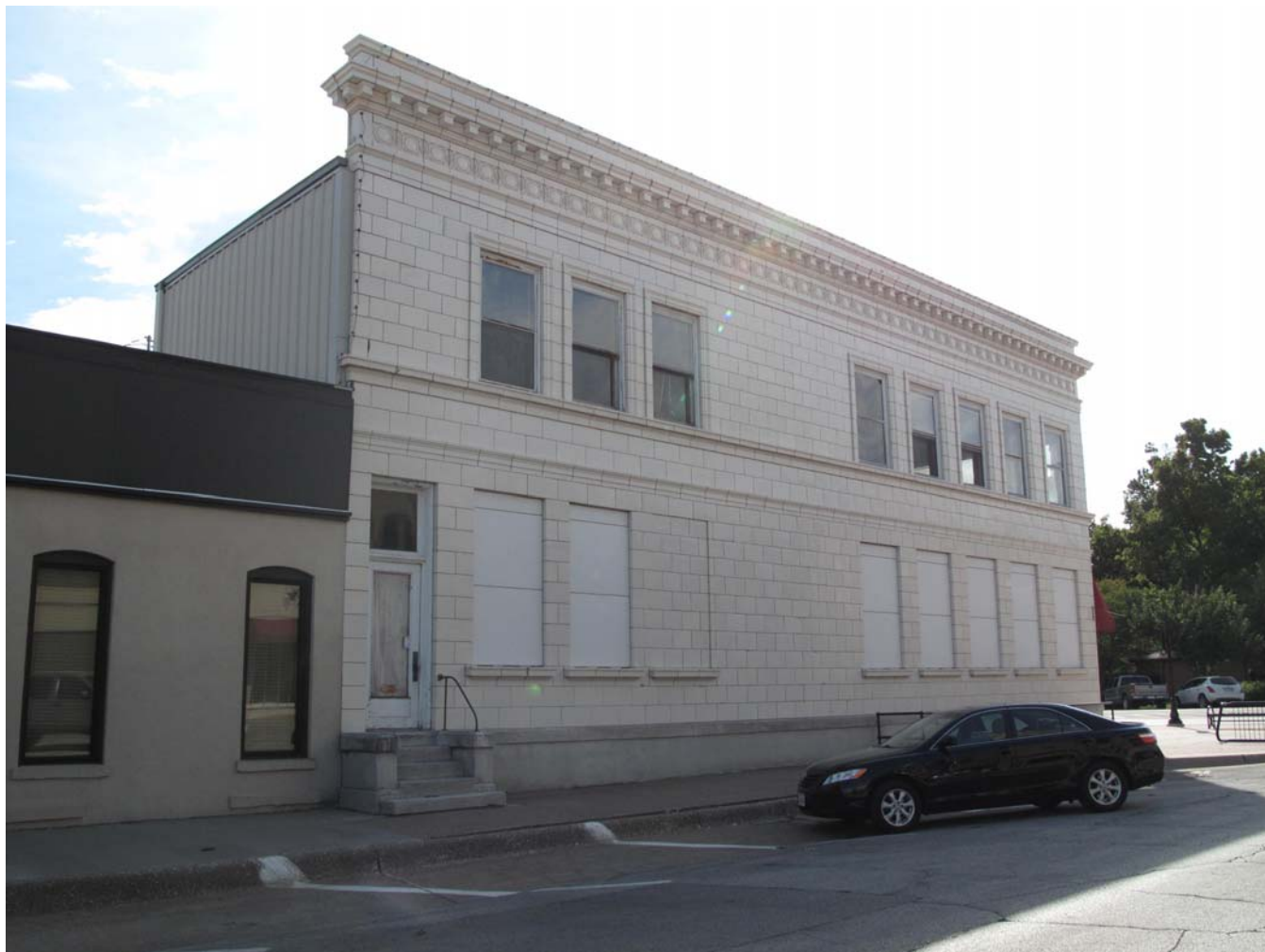
Photograph 92-00508-003 - North elevation, looking southwest (McCarley, September 20, 2011)
