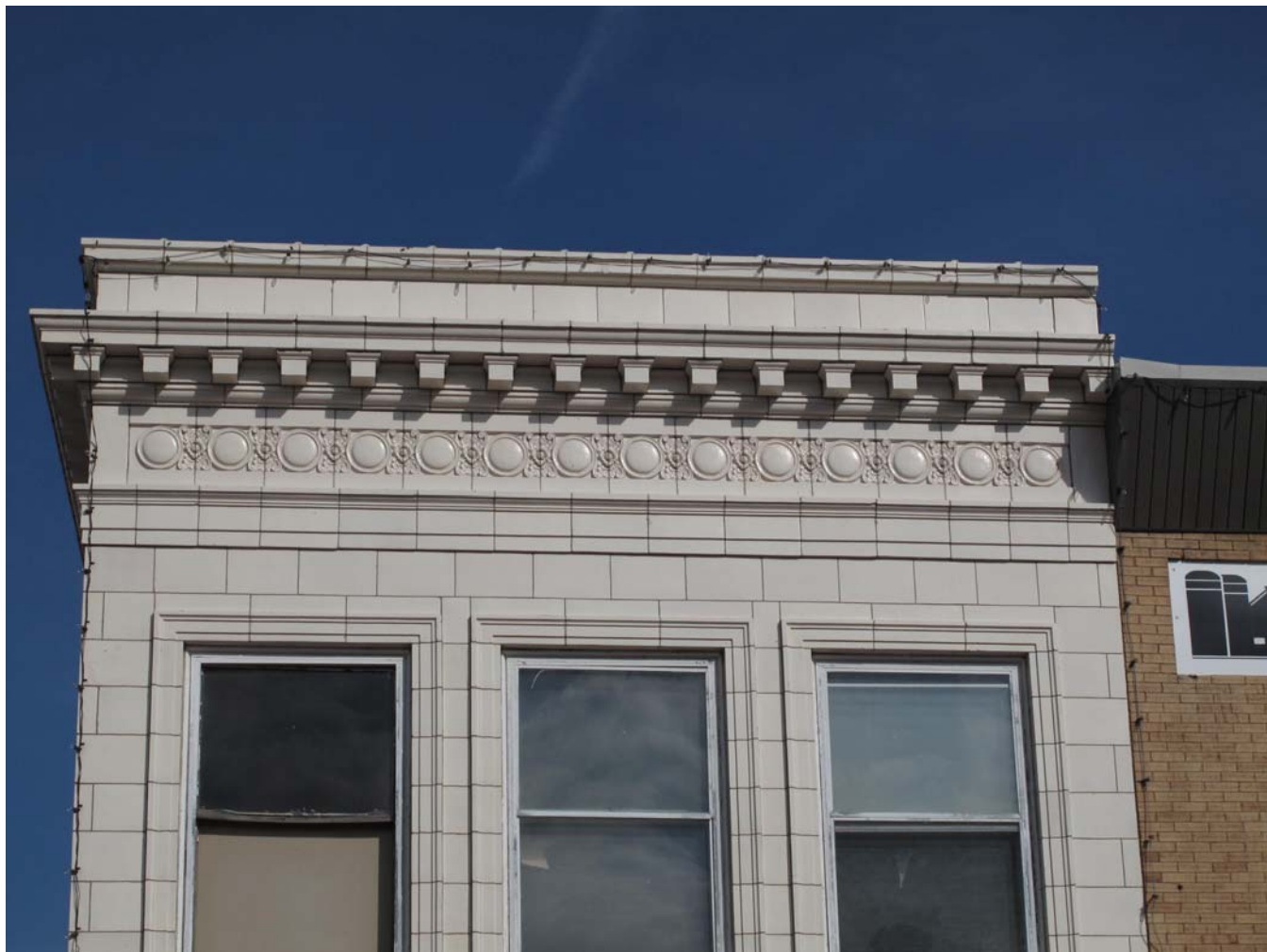
Photograph 92-00508-002 - Detail on west elevation, looking east (McCarley, September 20, 2011)
