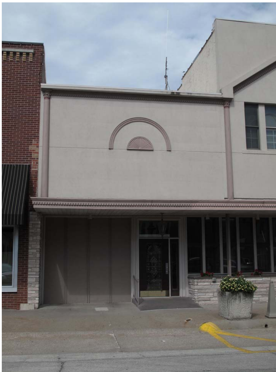
Photograph 92-00535-001 - South elevation, looking north (McCarley, September 20, 2011)
